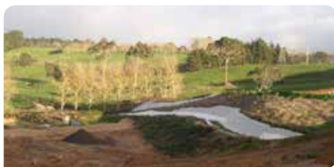
One of the many environmental controls in place along the Expressway
