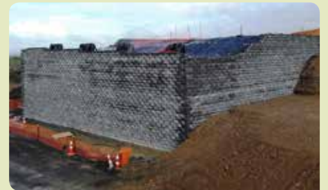
MSE wall being constructed at the Te Kauwhata Interchange
