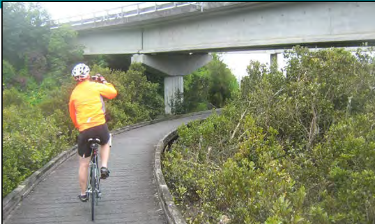
Existing timber boardwalk
