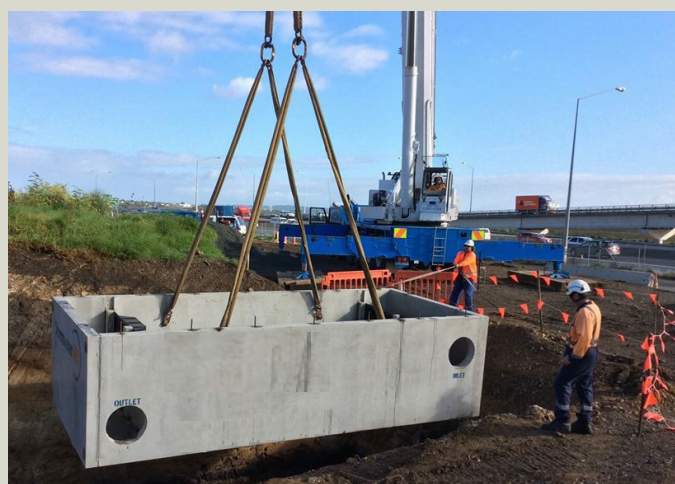
Underground stormwater treatment device being installed
