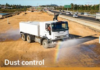
You may have noticed trucks driving along the construction areas spraying water. These water carts have an important job to dampen down dust coming from our site to prevent a possible hazard to passing motorists and cyclists. Due to the hot, dry summer weather we have several water carts all busy 'watering' different areas of the site.
