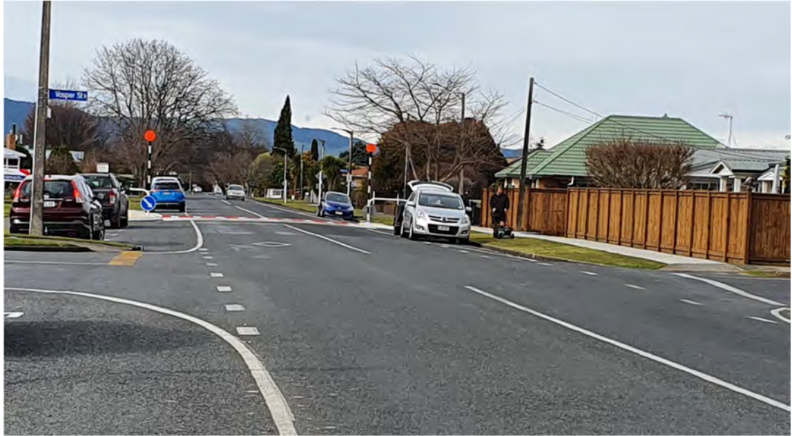
Figure 9 Raised safety platform west of Vosper Street.
