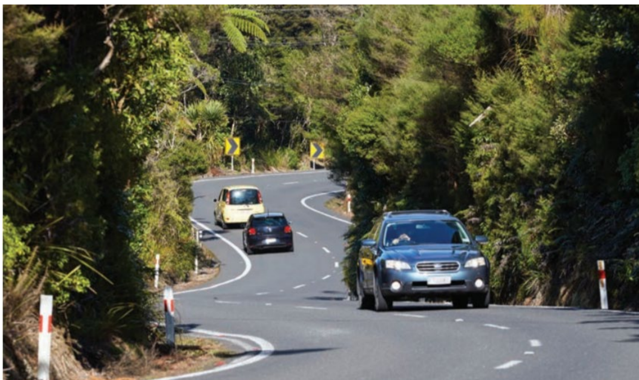
Figure 16 Example of Unforgiving Roads and Roadsides – State Highway Network
