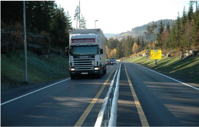
Figure 6: A narrow Norwegian 10m wide road with a steel median barrier.
