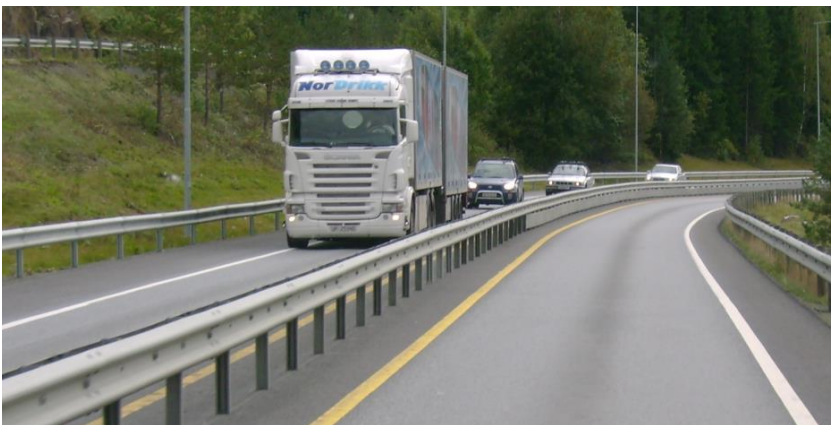
Figure 7: A wider cross-section Norwegian road with 3 steel barriers
