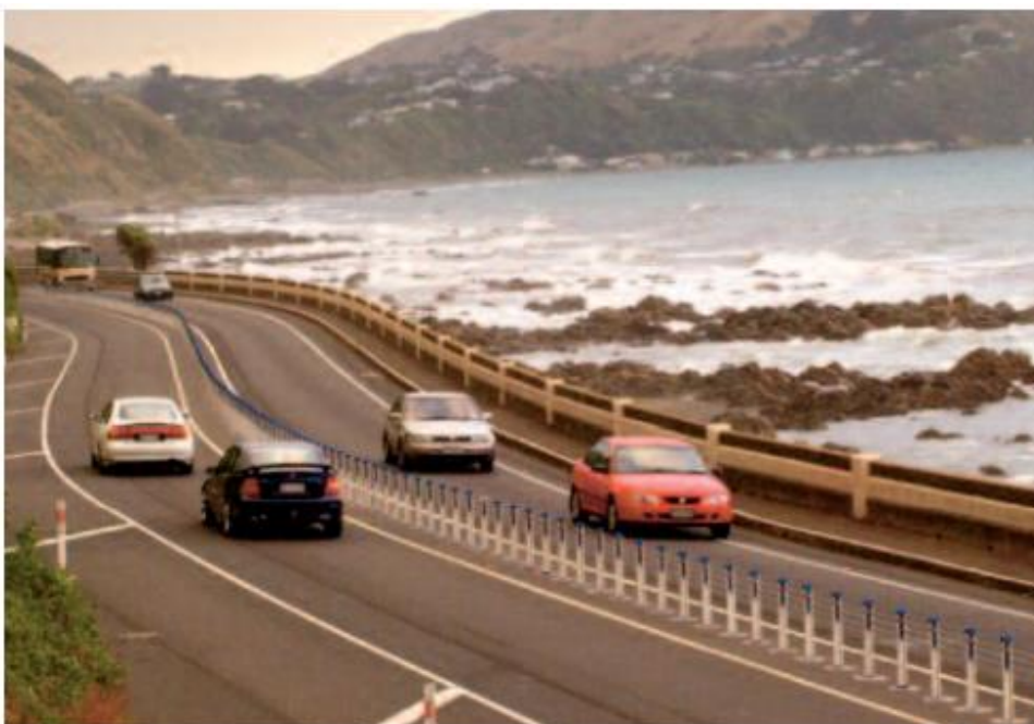
Figure 13: Narrow median wire rope barrier installation on Centennial Highway
