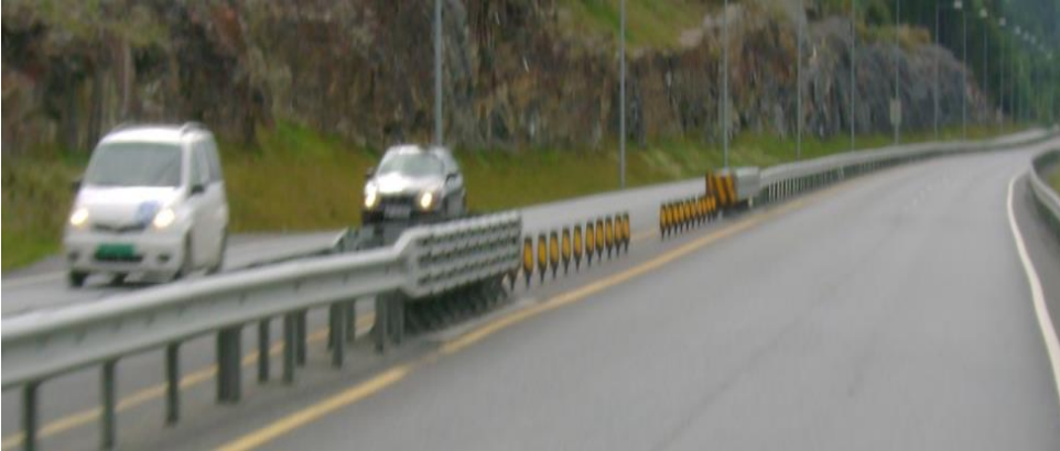
Figure 21: emergency turning facility on a steel barrier divided Norwegian road.
