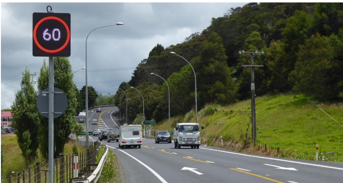
Figure 1: Northbound VSL sign at Brynderwyn Intersection Speed Zone
