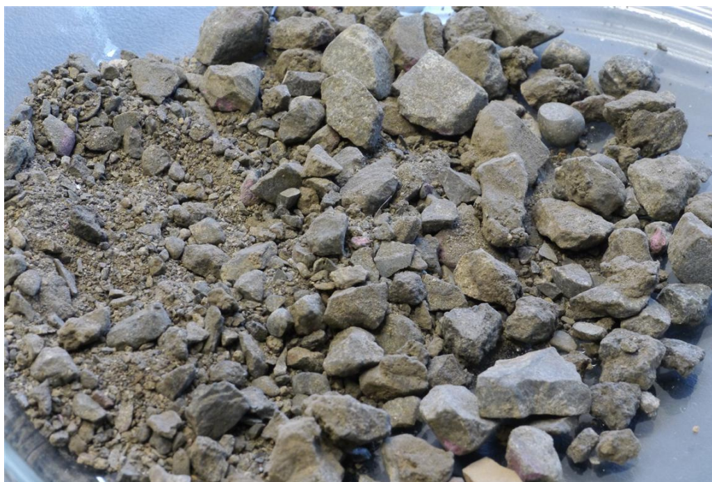
Figure 1: Aggregate extracted from a multi-layer chip seal core showing aggregate wear.
