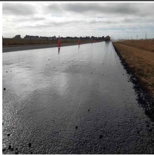
After application of 1 st coat of emulsion.
