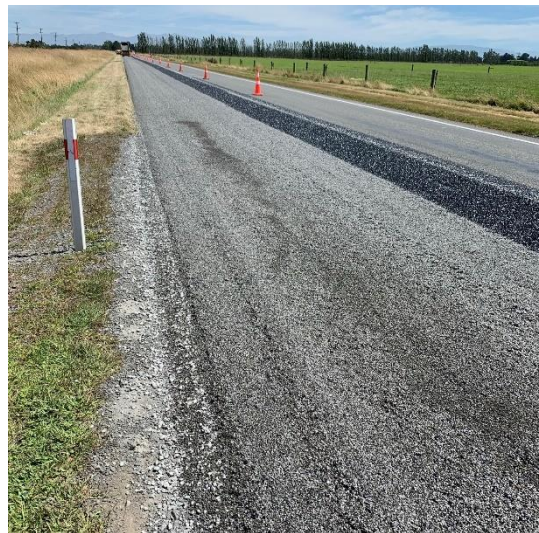
Grade 6 applied to left half of lane. Taken at 1216h.
