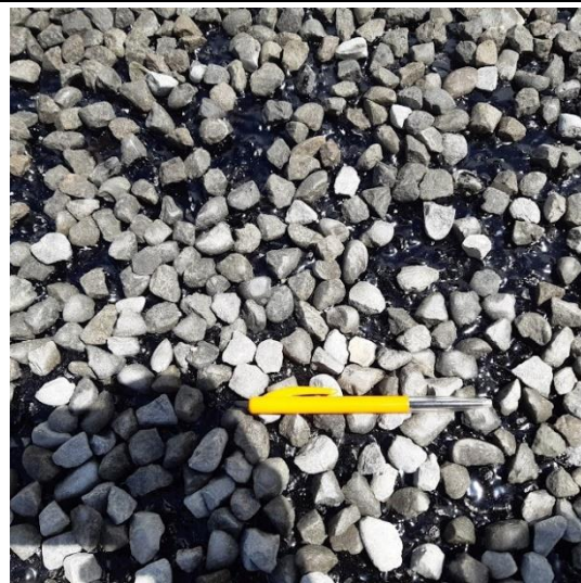
After application of grade 2 chip.
