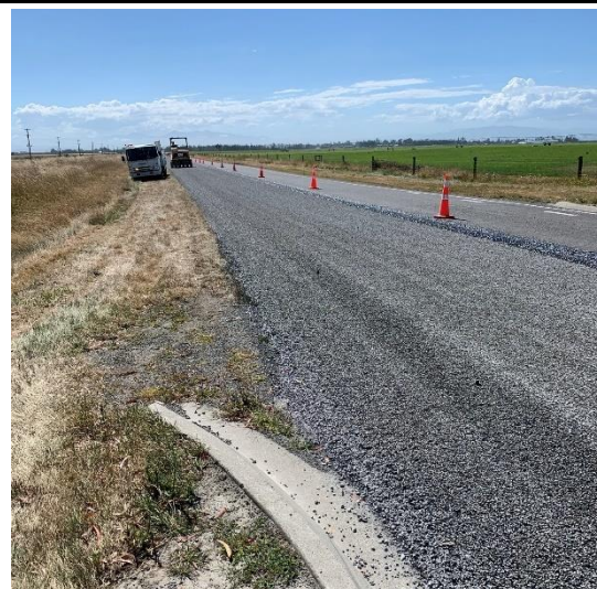
Rolling the grade 5 chip. Taken at 1614h.
