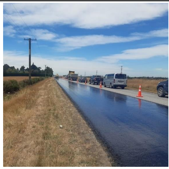
1 st coat of emulsion.
