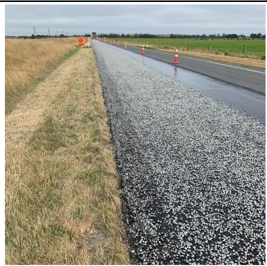
Application of grade 2 chip. Taken at 0905h.
