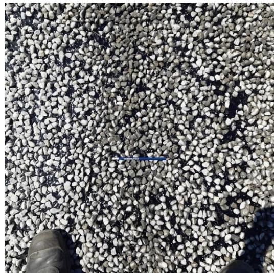
After application of grade 2 chip.
