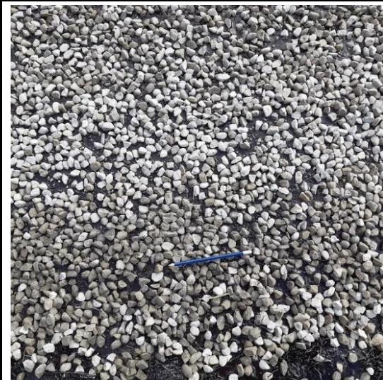
After application of grade 2 chip.
