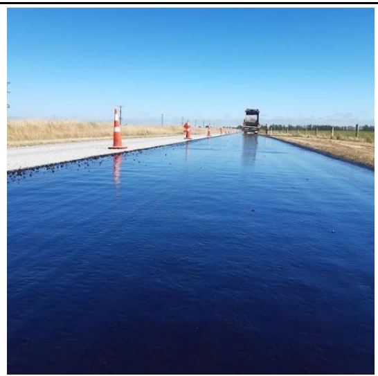
After application of 1 st coat of emulsion.
