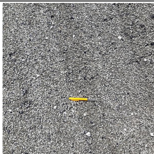
After application of grade 6 chip.
