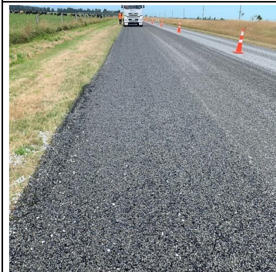
Application of grade 4 chip. Taken at 1550h.
