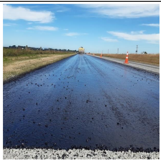
Application of 1 st emulsion coat.
