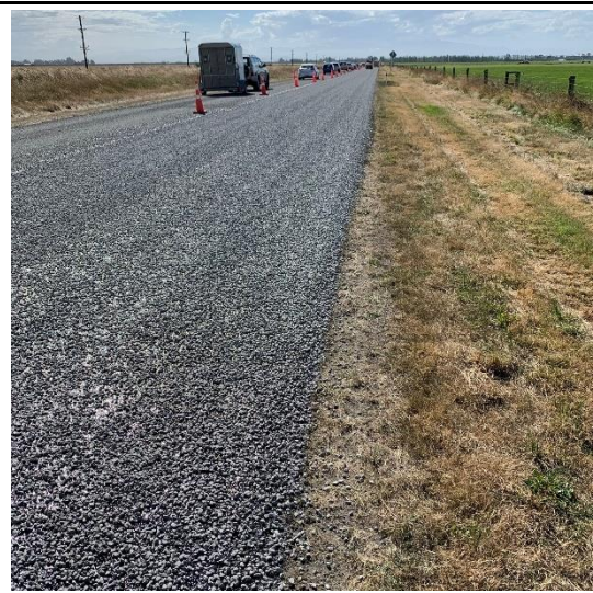
After application of grade 3 chip. Taken at 1705h.
