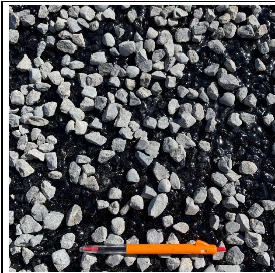
After application of grade 3 chip. Taken at 1704h.
