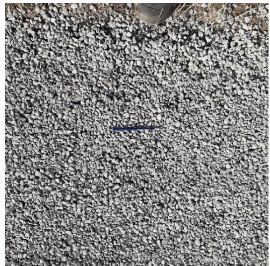
After application of grade 4 chip.
