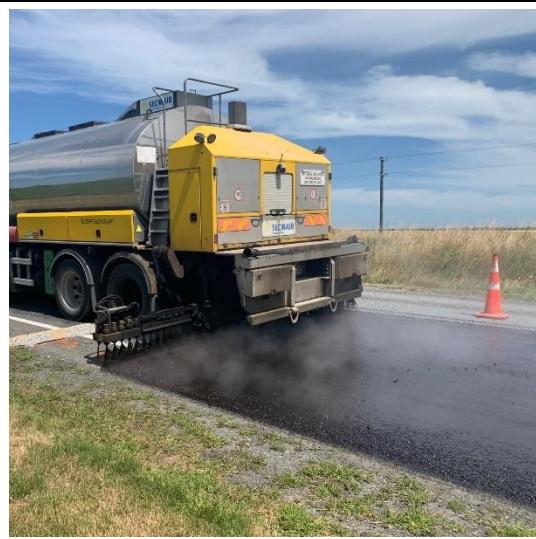
Applying 1 st coat of emulsion. Taken at 1453h.
