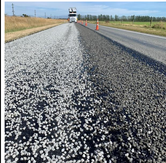
Grade 2 applied to right half of lane. Taken at 1047h.
