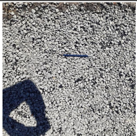
After application of grade 4 chip.
