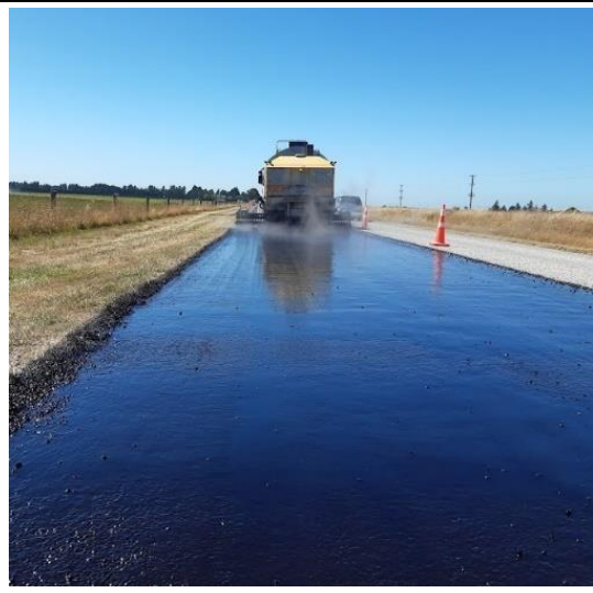
1 st coat of emulsion.
