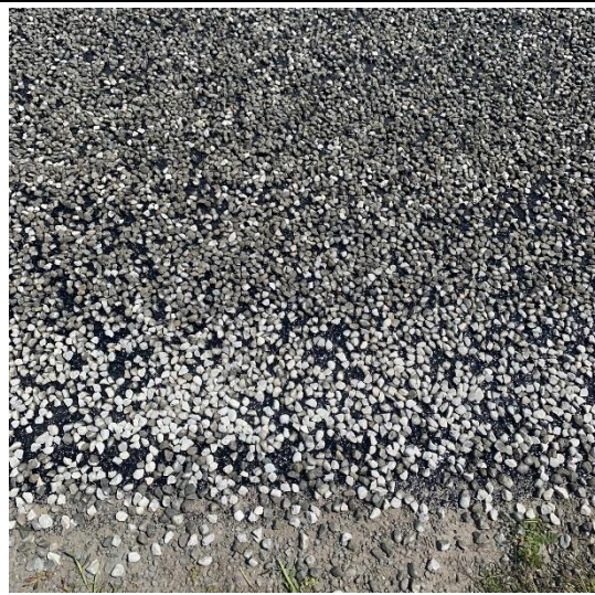
After application of grade 2 chip. Taken 1456h.
