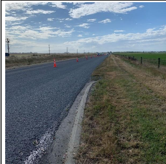
After application of grade 5 chip. Taken at 1800h.
