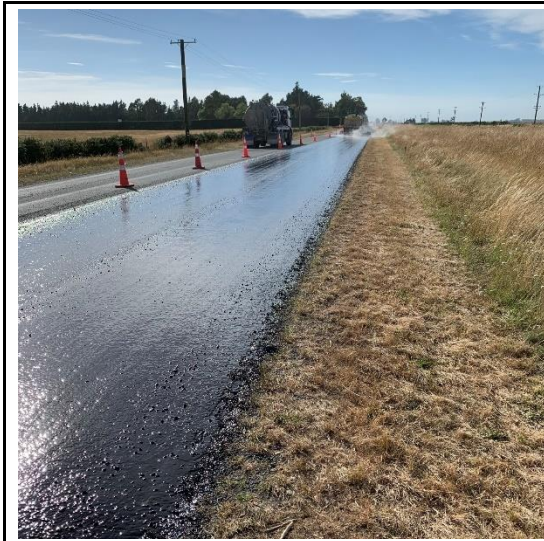
1 st coat of emulsion. Taken at 0918h.
