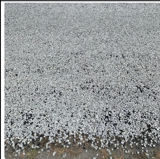
After application of grade 3 chip. Taken at 1306h.
