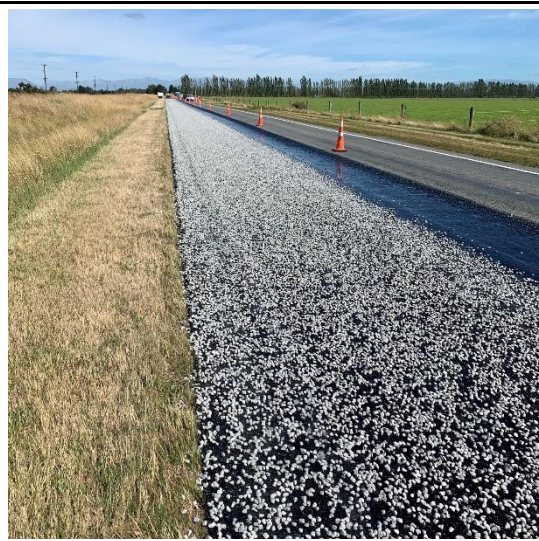
Grade 2 applied to left half of lane. Taken at 1045h.
