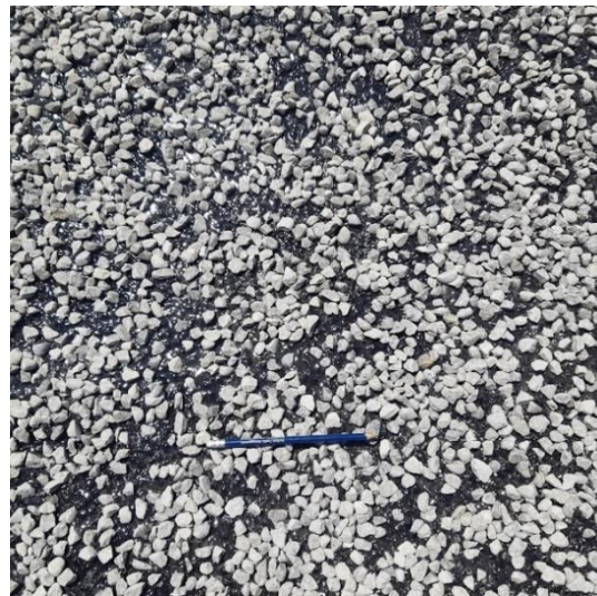
After application of grade 3 chip.
