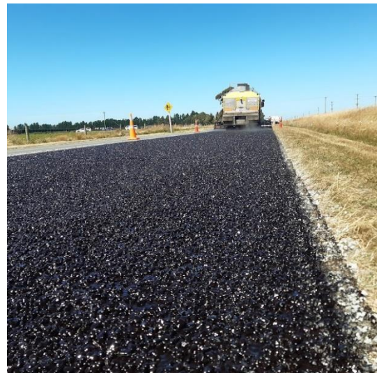
After 2 nd coat of emulsion.
