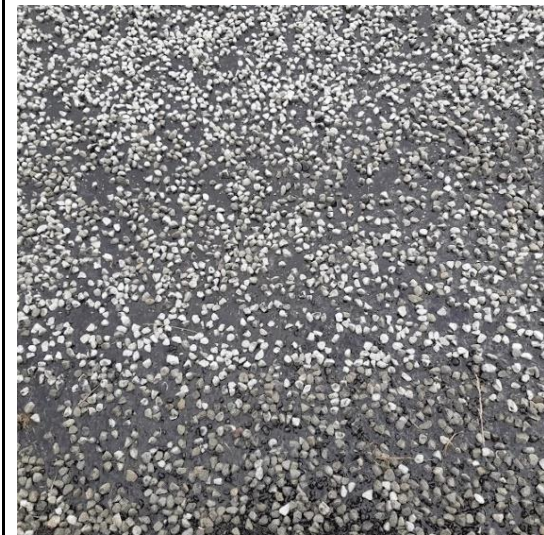
After application of grade 2 chip.
