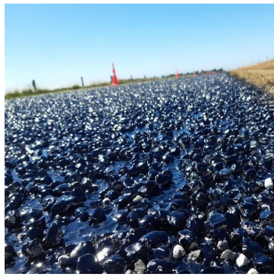
After application of 2 nd coat of emulsion.
