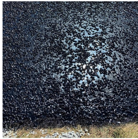
After application of 2 nd coat of emulsion. Taken at 1141h.
