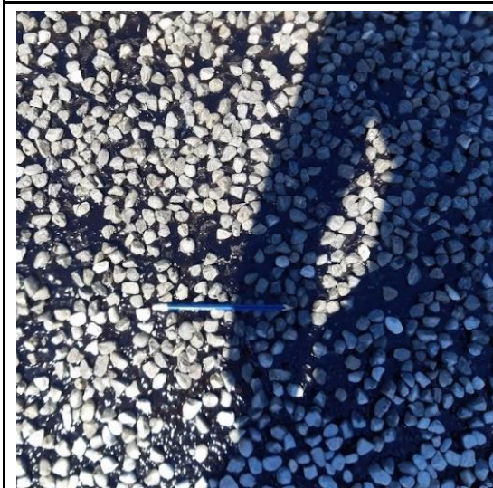
After application of grade 2 chip.
