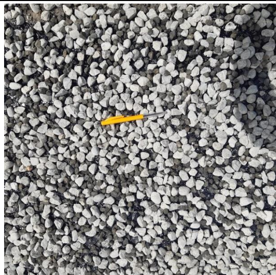
After application of grade 4 chip.
