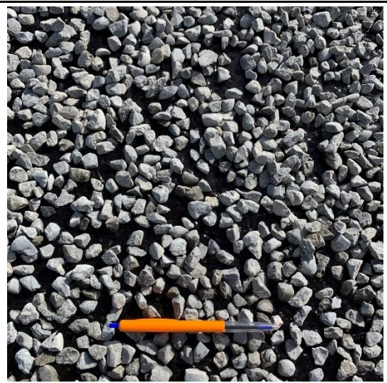
After application of grade 3 chip. Taken at 0924h.
