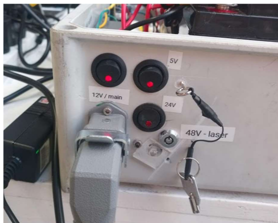
Figure 7: Switches and connections for power supply
