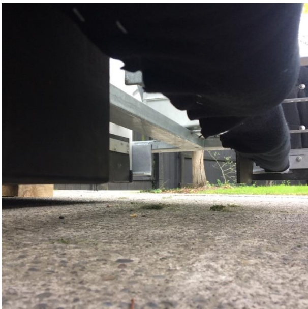
Figure 23 Section of inner rubber skirt removed
