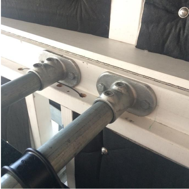
Figure 21 Steel mudguard tubes inserted into brackets
