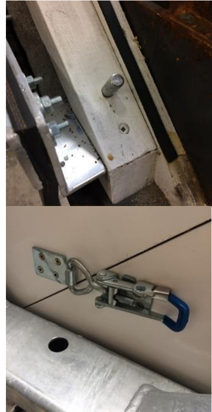
Figure 8 New pins and heavy-duty latches
