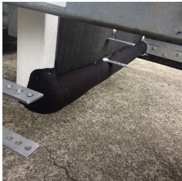
Figure 24 Felt-polyester layer added to lower timber member
