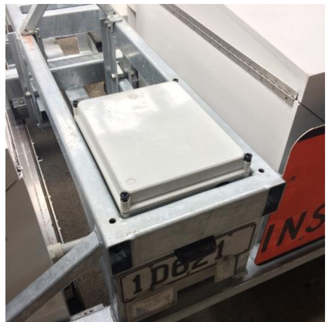
Figure 12 Separate battery enclosure can be removed for overnight charging
