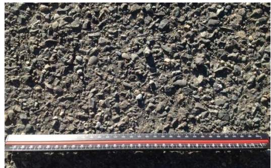
Location 2 – Two-coat chipseal
