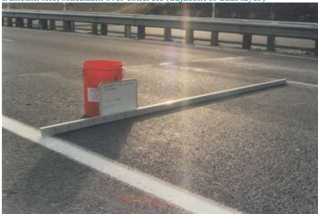
Dunedin site, Macadam over concrete (adjacent to dual layer)
