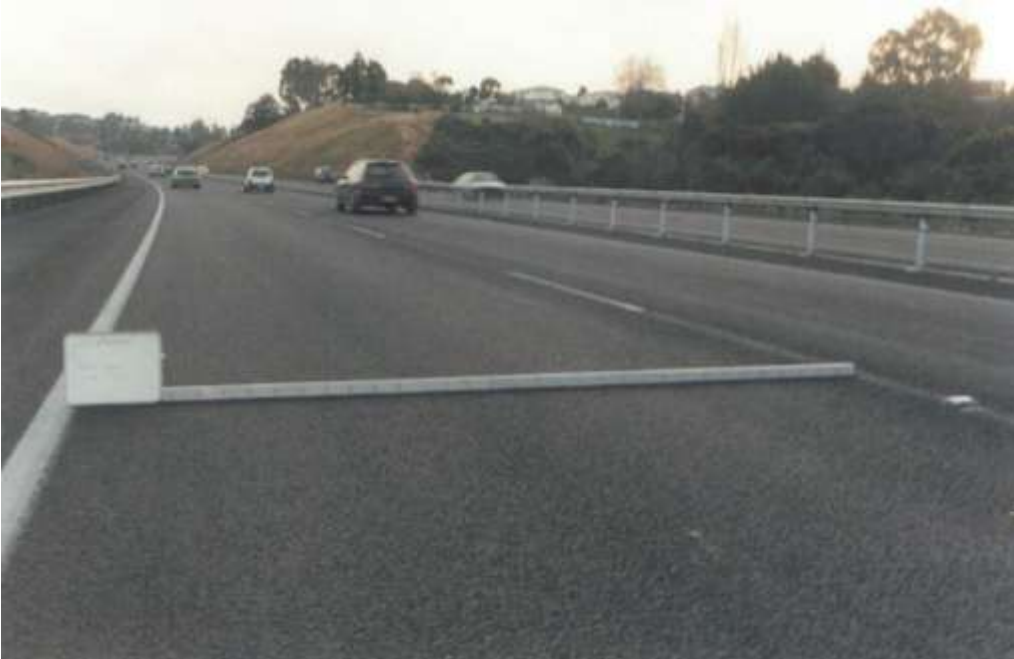
Dunedin site, ultra-thin asphalt Pavetex (adjacent to OGPA 14)
