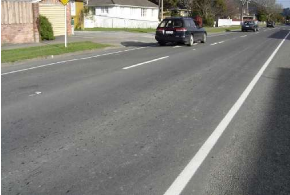
Lower Hutt, Wainui Road asphaltic concrete (note cracking)
