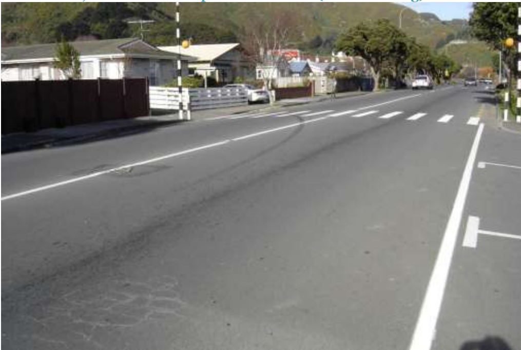
Lower Hutt, Wainui Road asphaltic concrete (note cracking)
