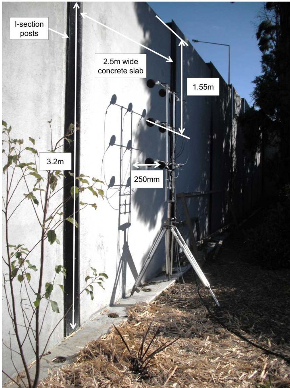
Figure E.3 Composition of the concrete traffic noise barrier, test setup during an element measurement
