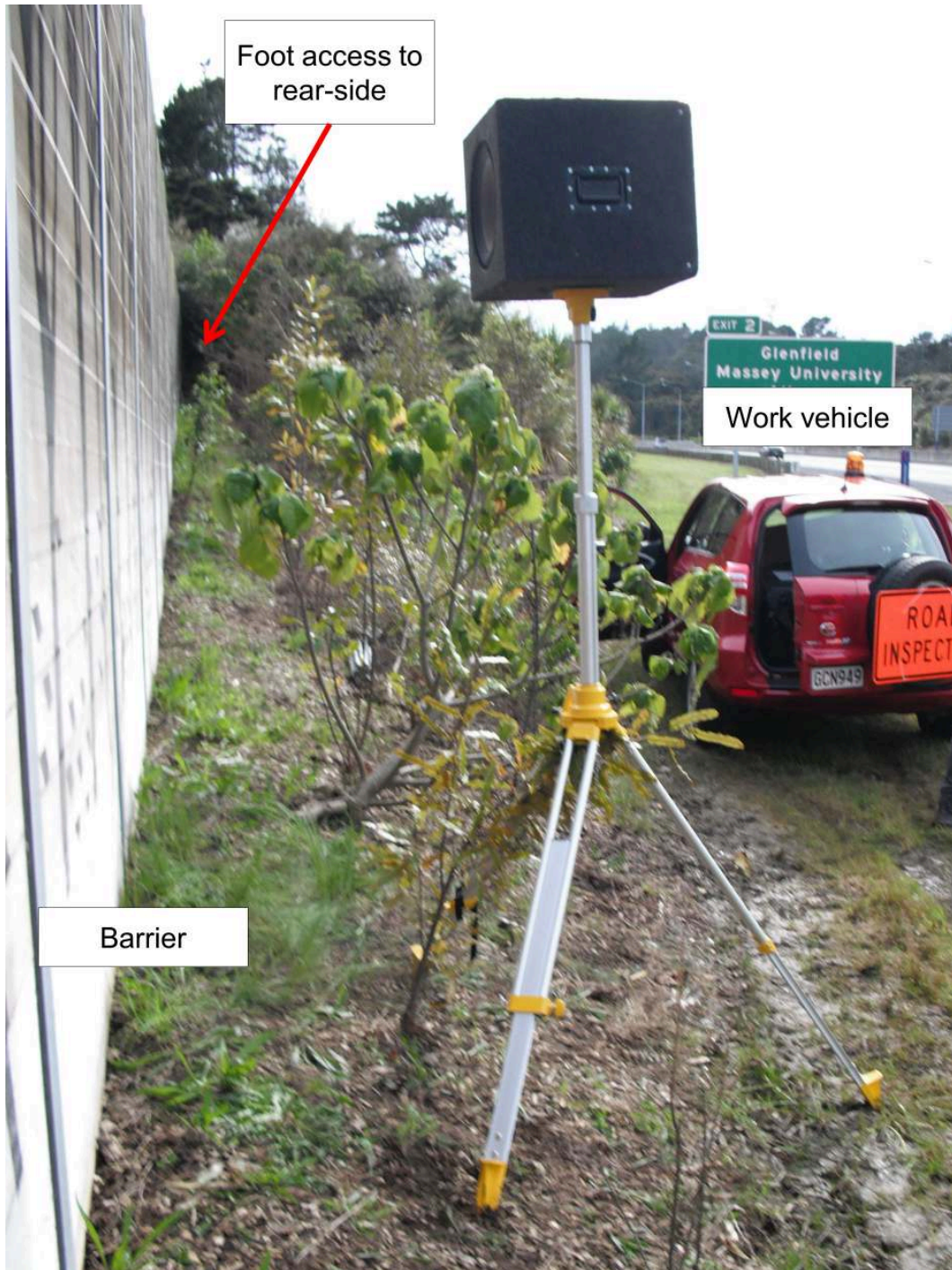
Figure 3 Road inspection site layout, Greenhithe
