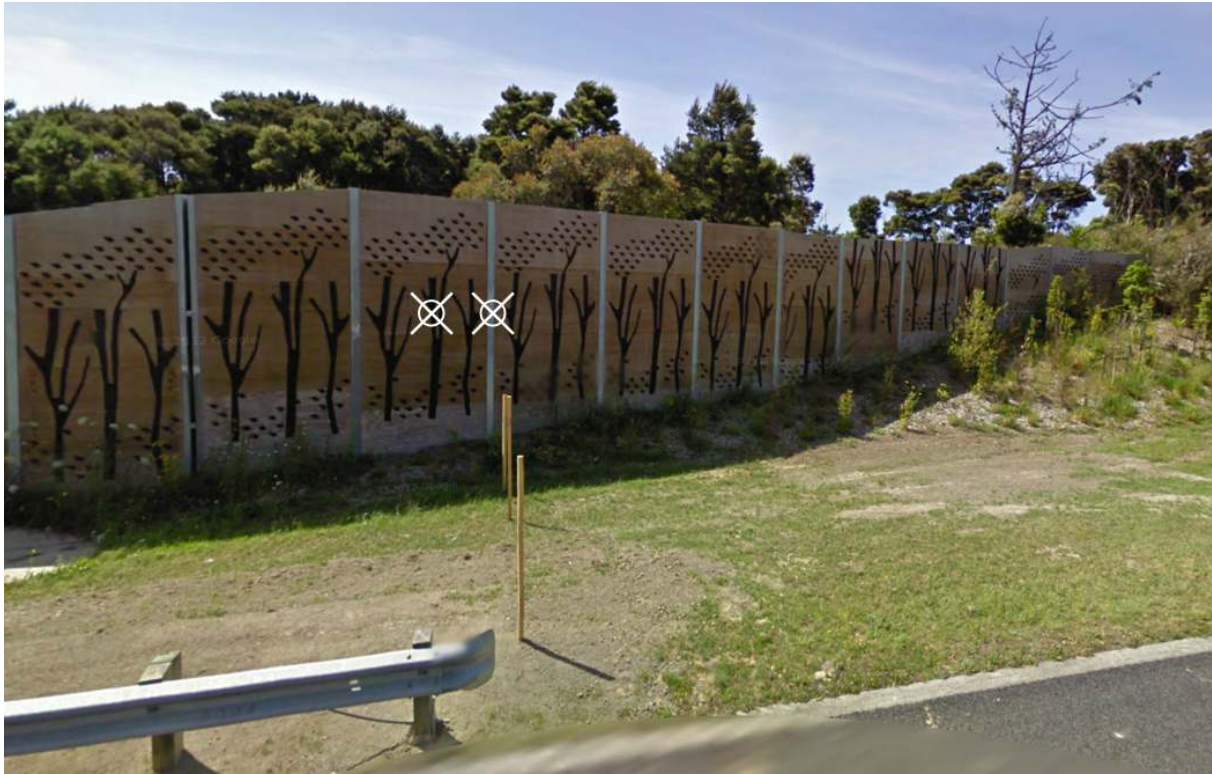
Figure C.1 General view of the traffic noise barrier under test (road-side), the crosses mark the measurement positions. Image from Google Maps
