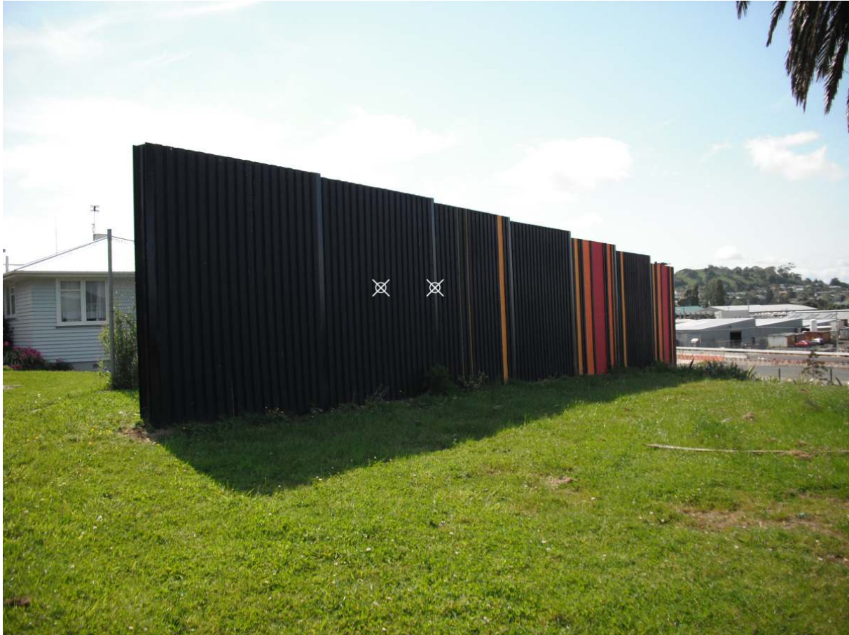
Figure D.1 General view of the traffic noise barrier under test (road-side), the crosses mark the measurement positions
