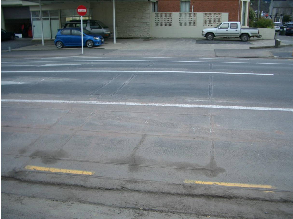
Figure F1 Photograph of Traffic Sensors on SH1 at Duke Street Intersection
