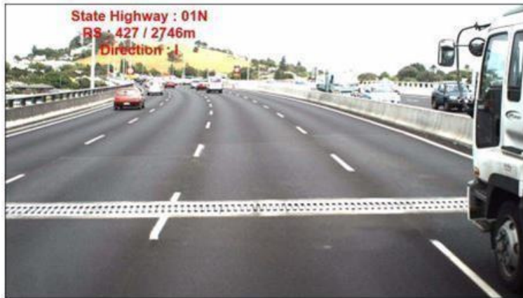
Figure 4-10 Mangere Bridge finger joint
