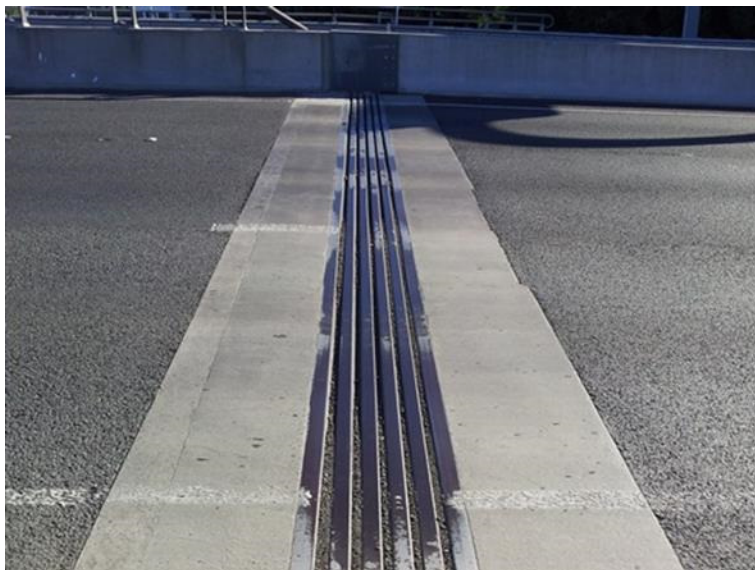
Figure 4-11 Tauranga Harbour Bridge modular joint
