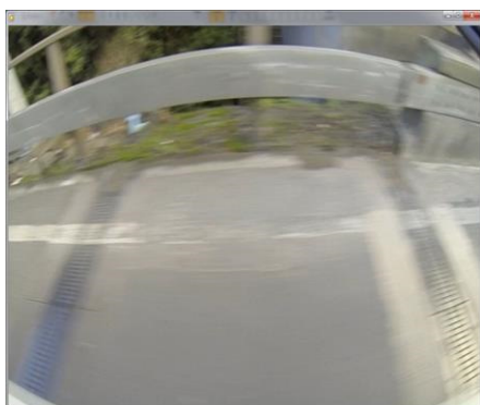
Figure 3-8 Photo of Clifton Terrace bridge joint taken from test vehicle at a speed of 80 km/h
