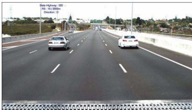
Figure 4-10 Mangere Bridge finger joint
