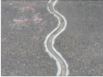
Figure 2-3 Wave shaped joint (Maurer Sohne)
