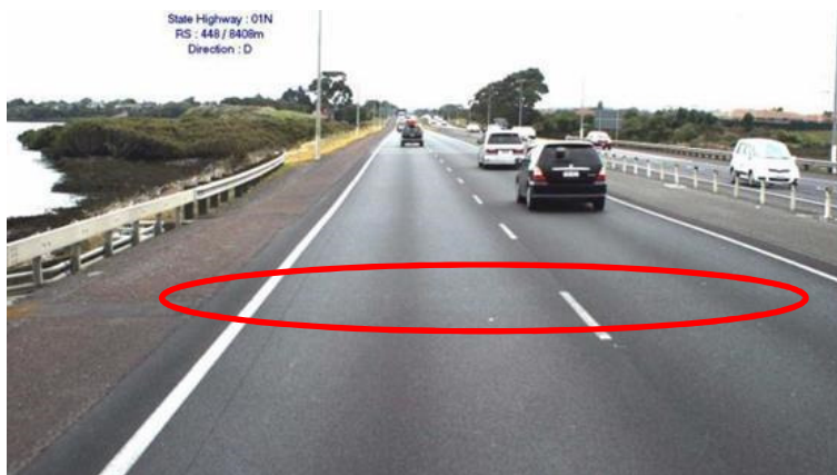
Figure 4-4 Air gap joint covered by road surface
