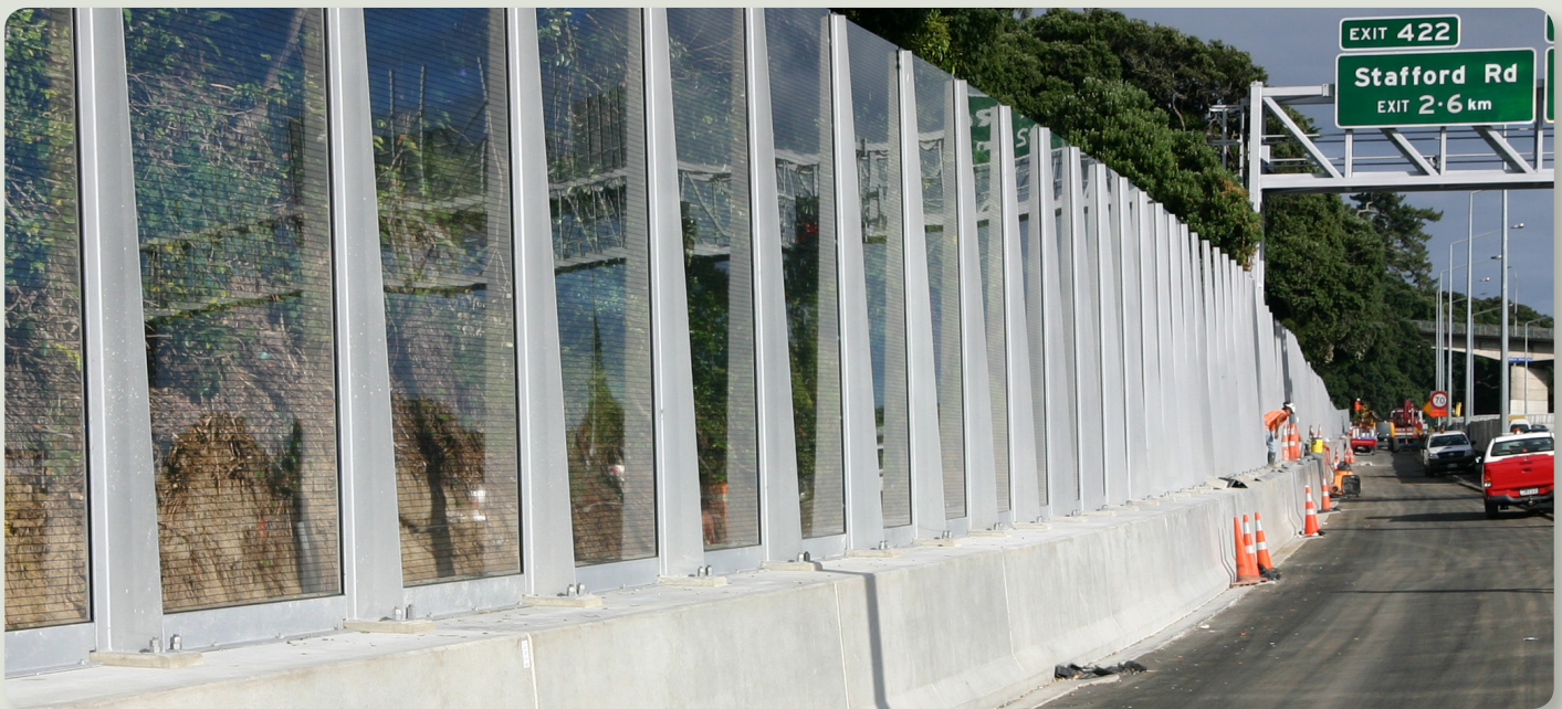
The projecting tees of the noise barrier support post were rotated to face the motorway side as a solution to help reduce the incidence of sunstrike.
