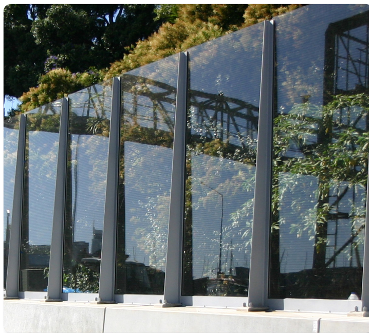
An analysis of transparent materials concluded that acrylic panels were best suited for this location, based upon the enhanced optical clarity of acrylic.
