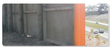
Construction issues are evident on this barrier: the rear of the barrier is unpanelled and unpainted, and gaps show between the barrier and the ground.
