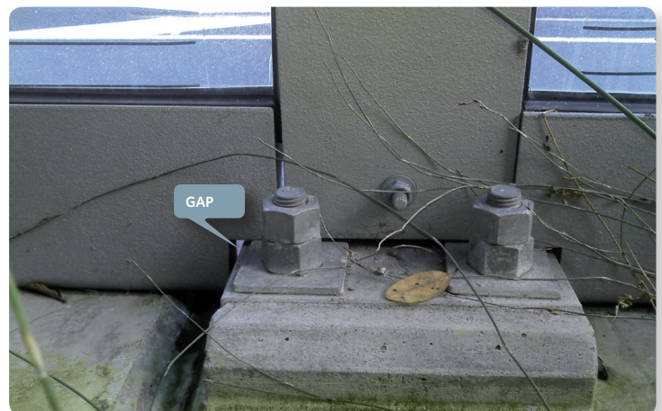
St Marys Bay acrylic noise barrier posts – the effects of small gaps can be investigated
