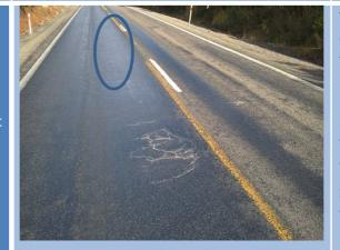
Yes this is an OPM defect. Treatment is too late and should be included in next year's program. Sandwich seal is appropriate treatment. Water cutting not required.
