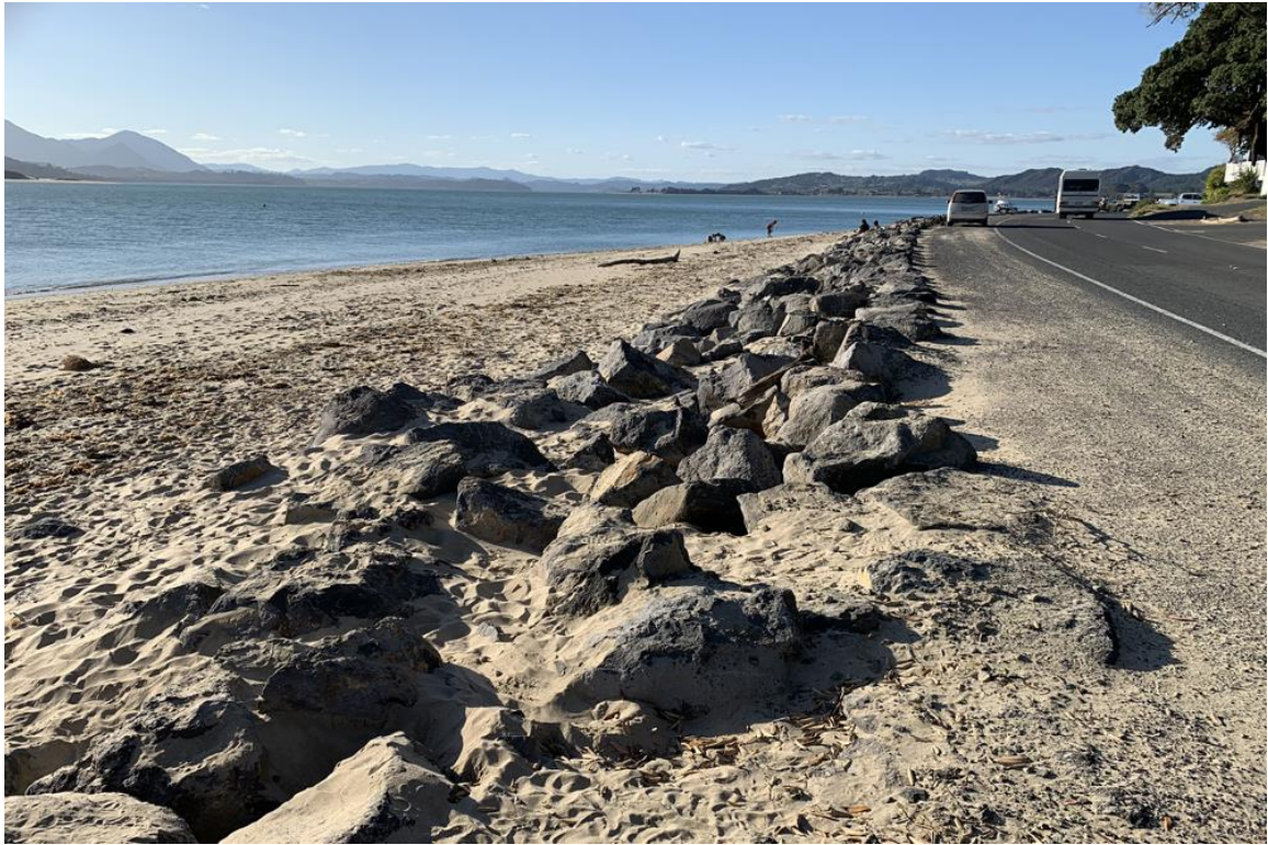
Figure 5: SH12 Looking south towards Opononi erosion protection in place (after)
