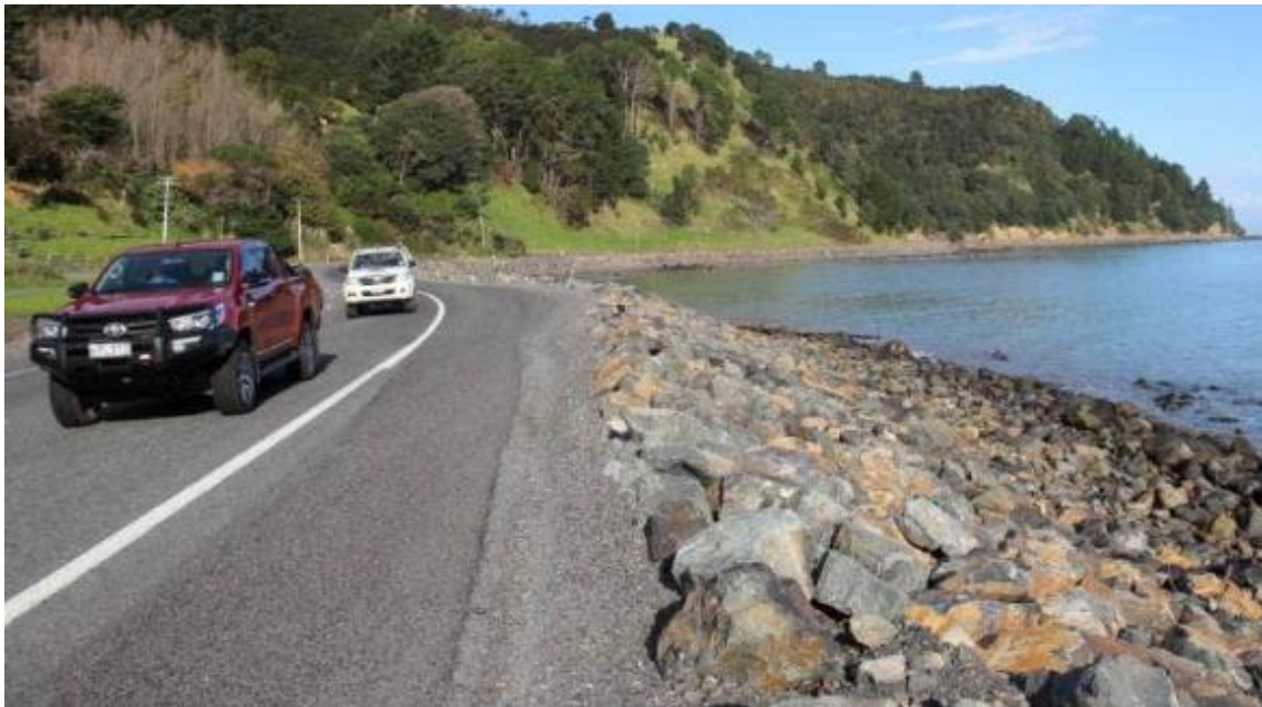
Figure 10: State Highway 25 (Firth of Thames Coromandel) sea wall repairs
