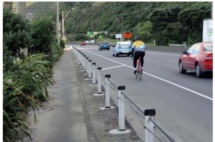
The existing cycle lane and walkway
