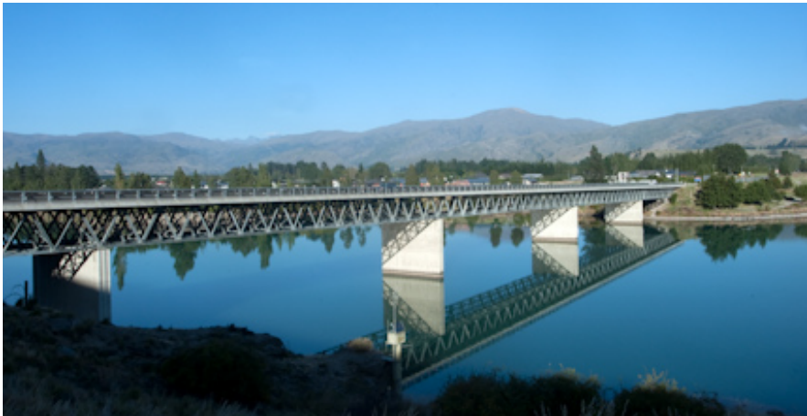
Bridge over Lake Dunstan
