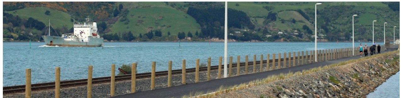
SH88 Dunedin to Port Chalmers walking & cycling path project
