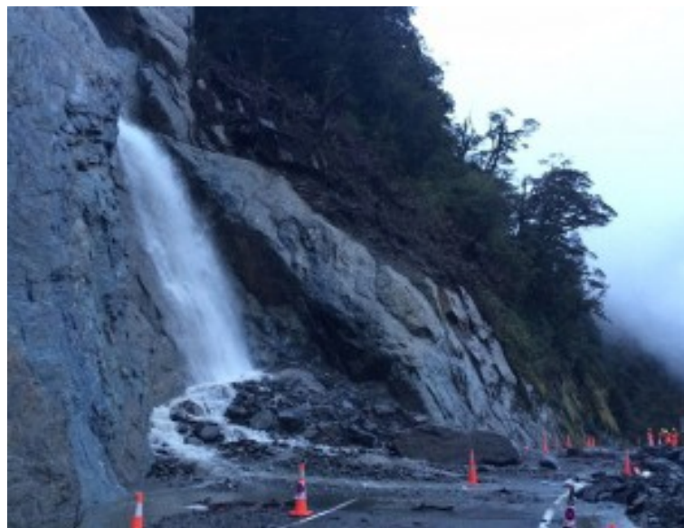
Large landslide closed State Highway 6 on the West Coast between Haast and Makarora in 2013
