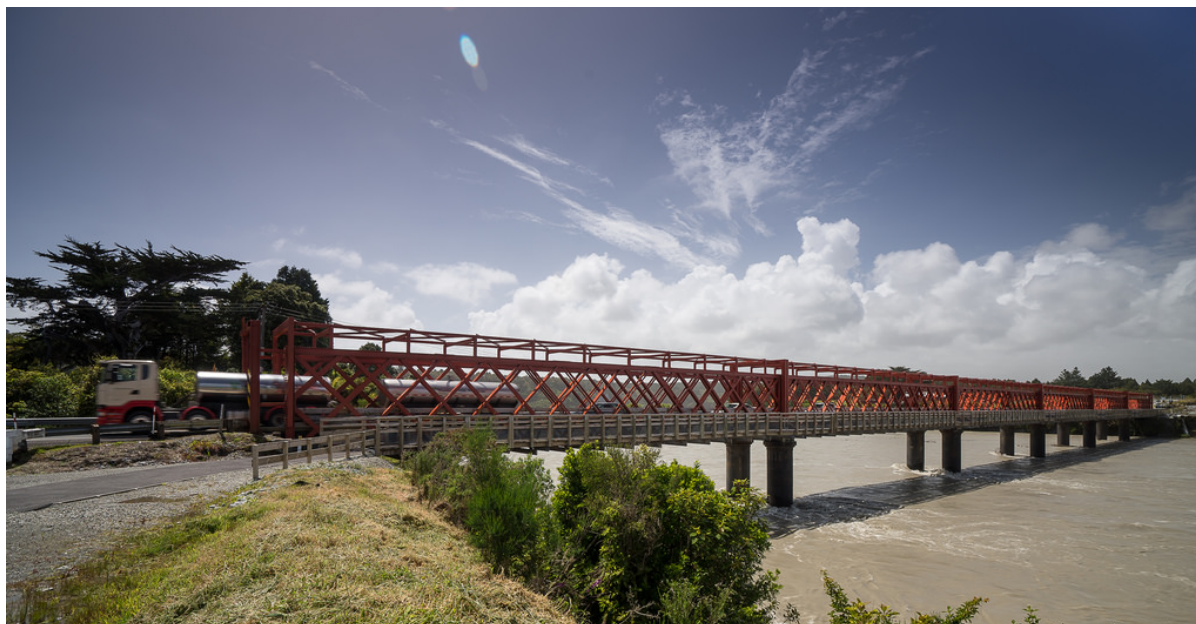
New Taramakau Bridge sod turning
