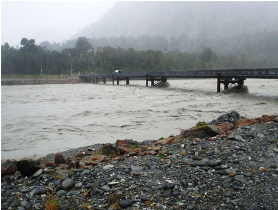
Flood water pouring under the SH6 Waiho River Bridge in south Westland
