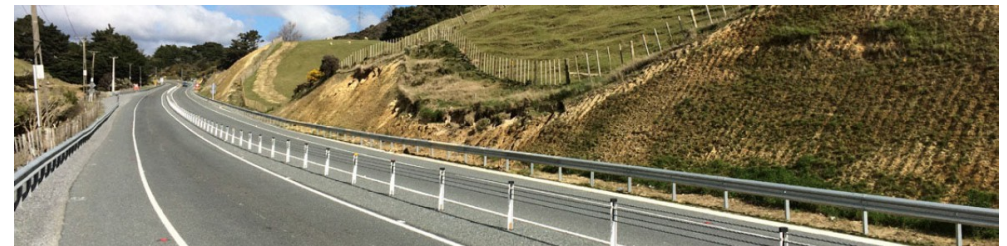
SH58 Safety improvements
