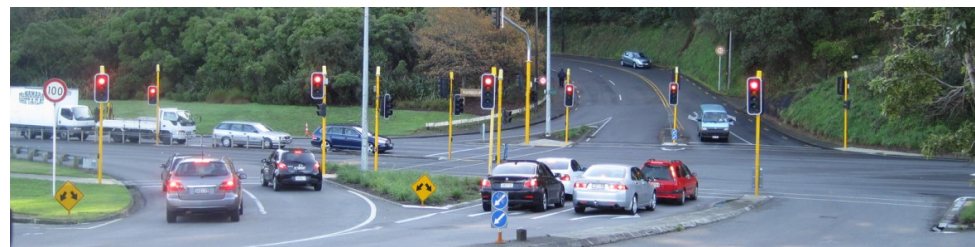
Looking at ways to reduce congestion and improve access and safety on State Highway 2 at the Melling & Block Road intersections
