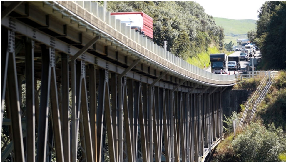
Mohaka River bridge is closely monitored
