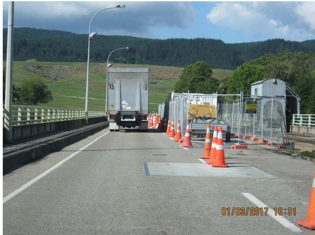
SH30 RP84 – Whakamaru Dam signalled bridge access
