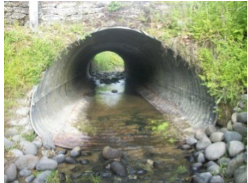
SH43 Nevins Hill culvert
