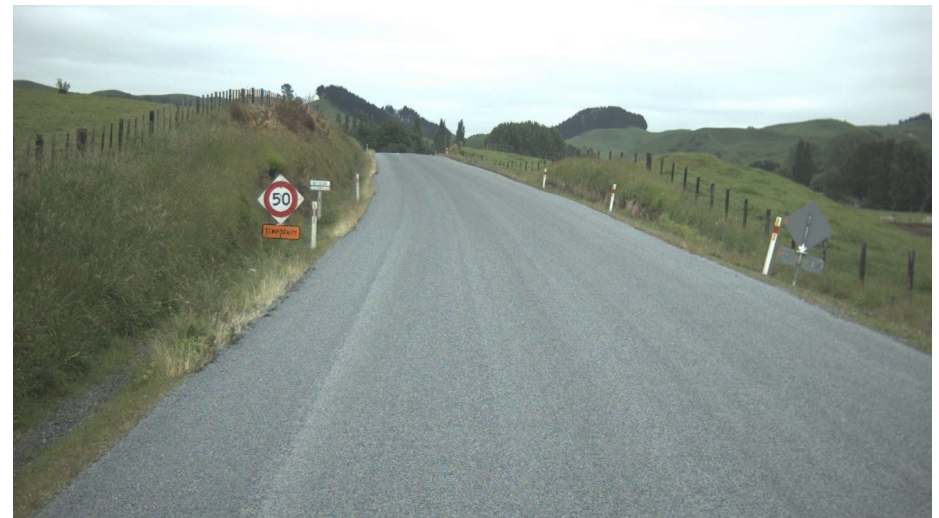
SH30 RPO resealing with 50km temporary speed limit
