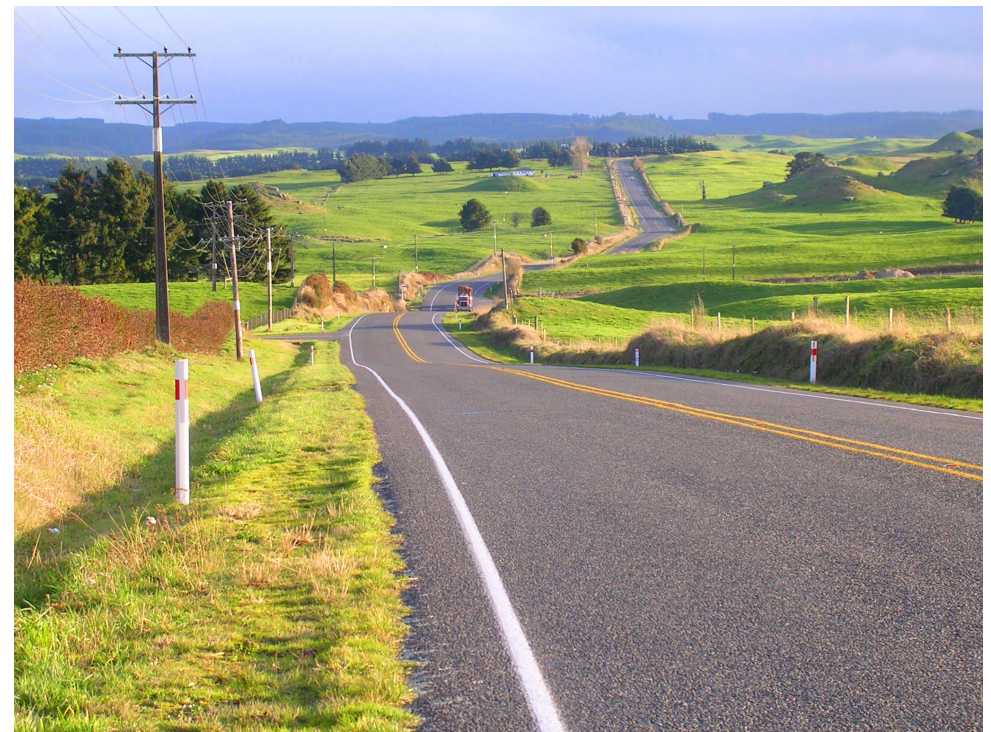
SH30 Whakamaru has low maintenance demands due to low traffic volumes
