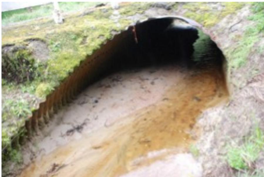
SH43 Awahou stream culvert
