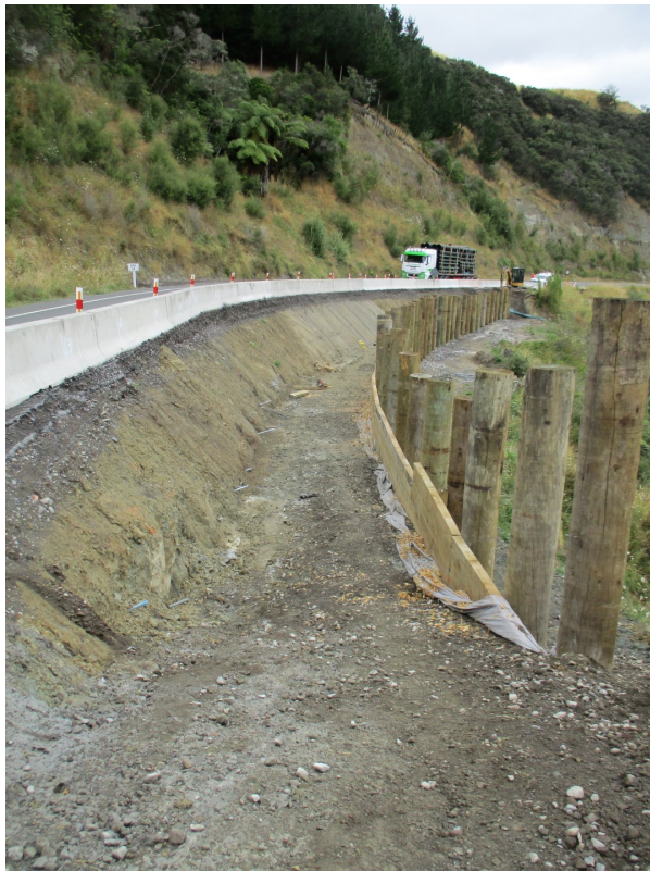
SH4 Storm Damage reinstatement works
