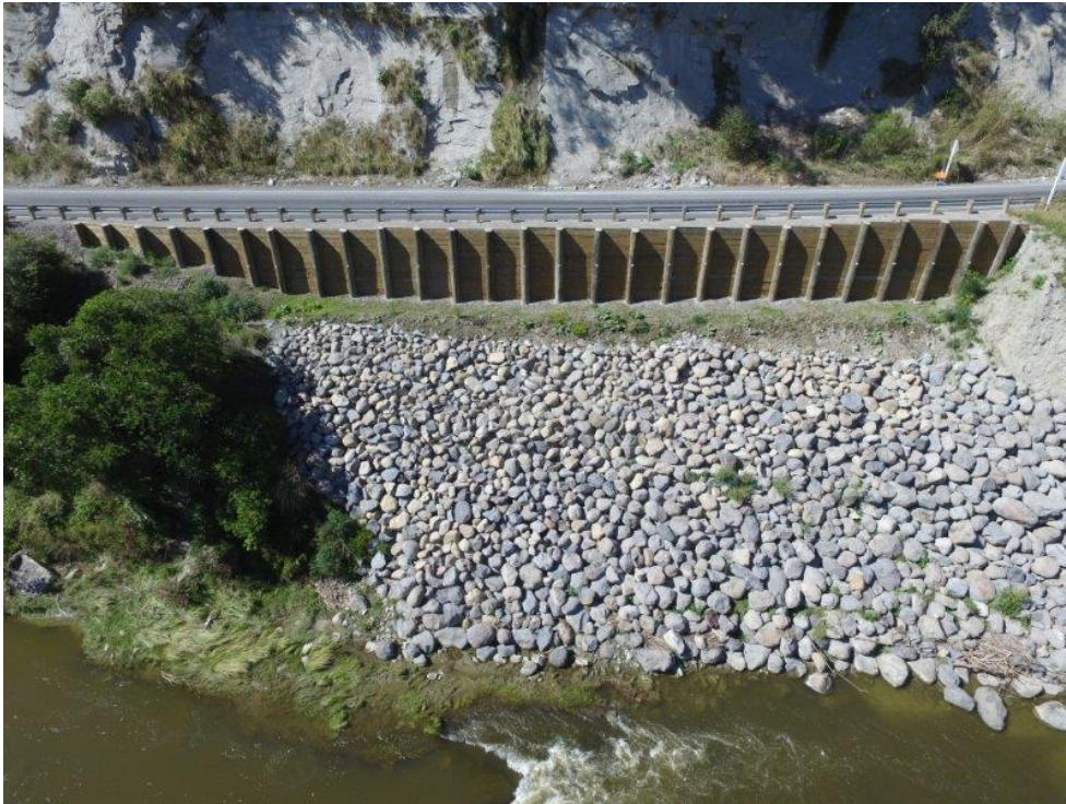
SH4, RP176, reinstatement post storm damage
