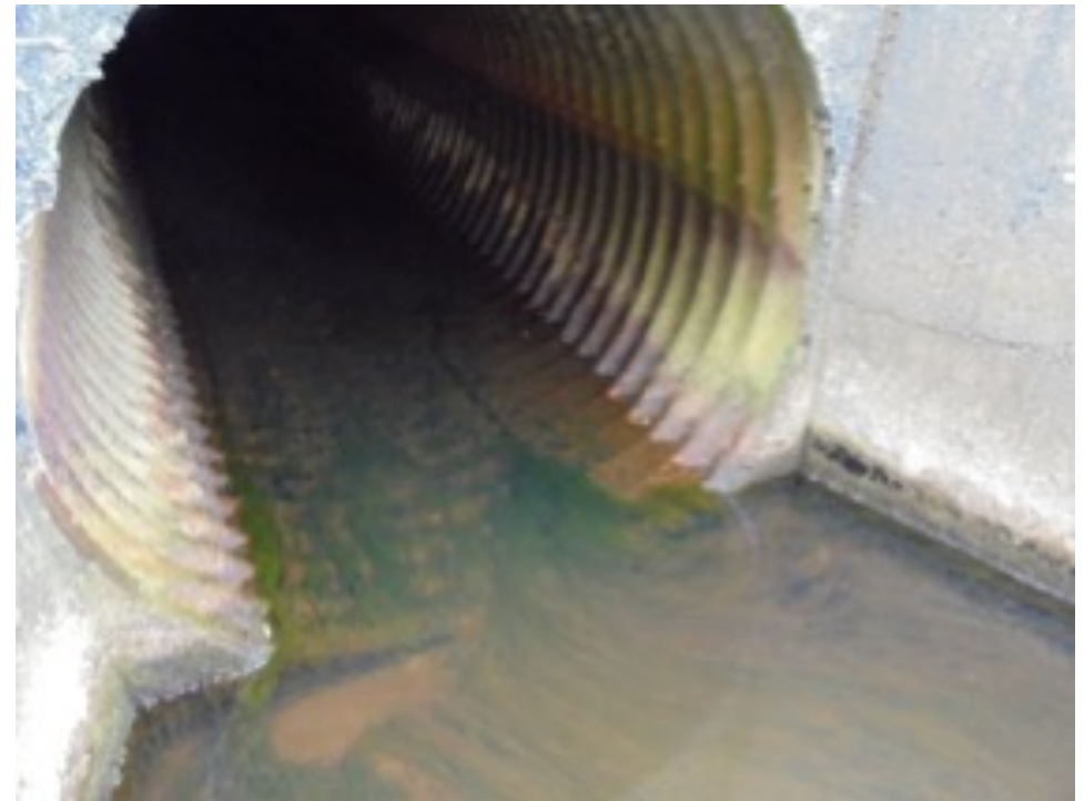
SH4 Steel culvert
