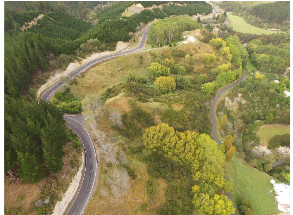
SH4 prone to erosion and undercut, particularly during storm events
