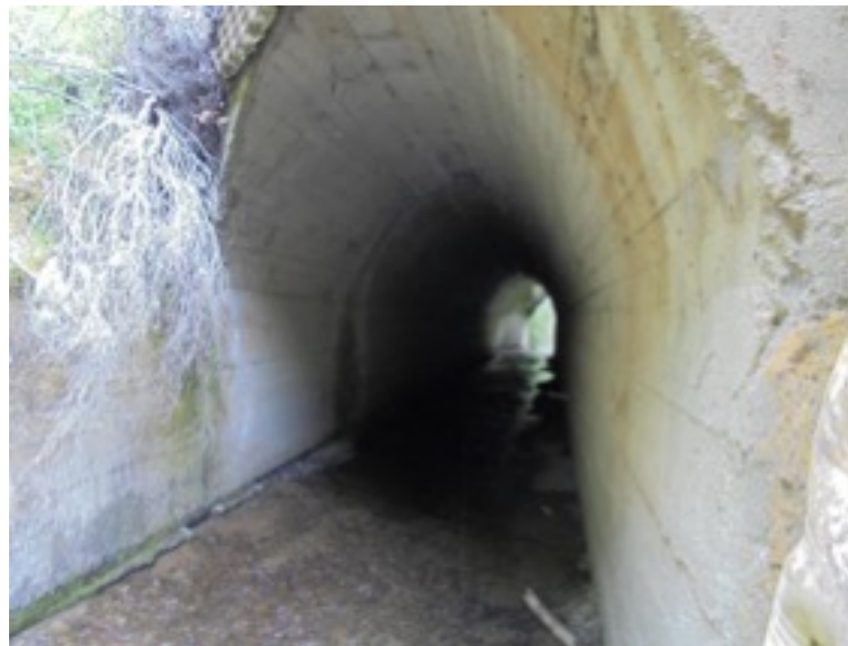
SH4 Pahihi Culvert, RP188
