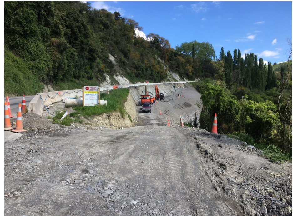
SH4, RP176. 2015 site 16 Storm Damage reinstatement works
