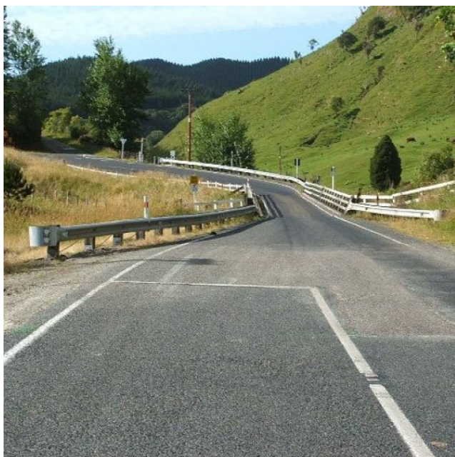
The Motu Bridge is a narrow, one-lane bridge with poor alignment on its approaches.
