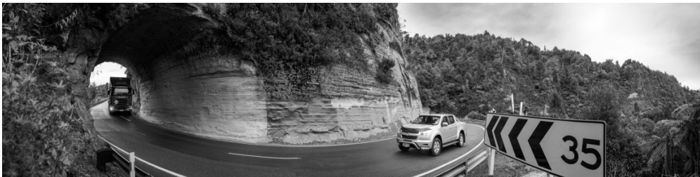
State Highway 3 (SH3) from Awakino Gorge to Mt Messenger to improve safety, resilience and route availability.
