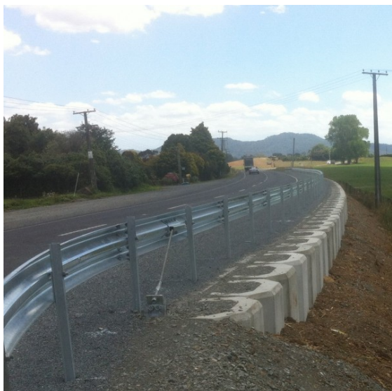
Taupiri safety improvements
