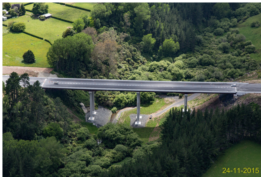
Waikato expressway – Karapiro Gully Viaduct
