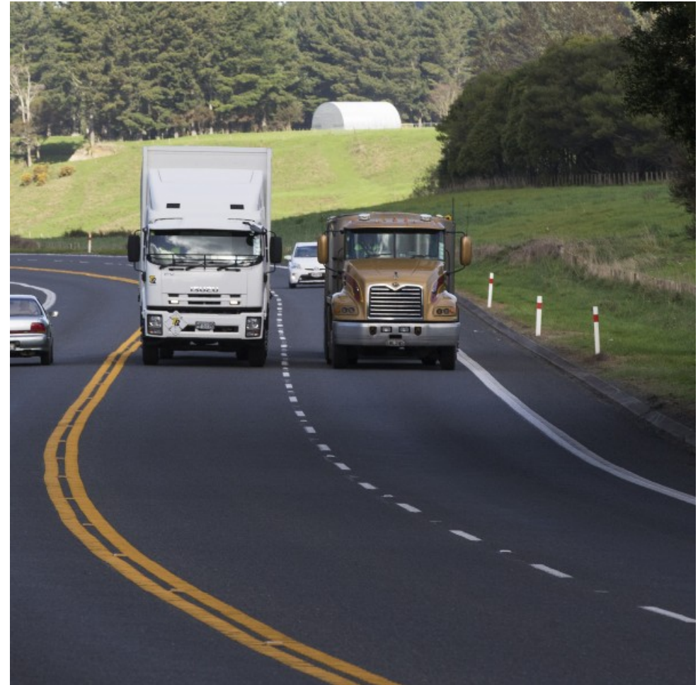
SH1 - Cambridge to Piarere safety improvements
