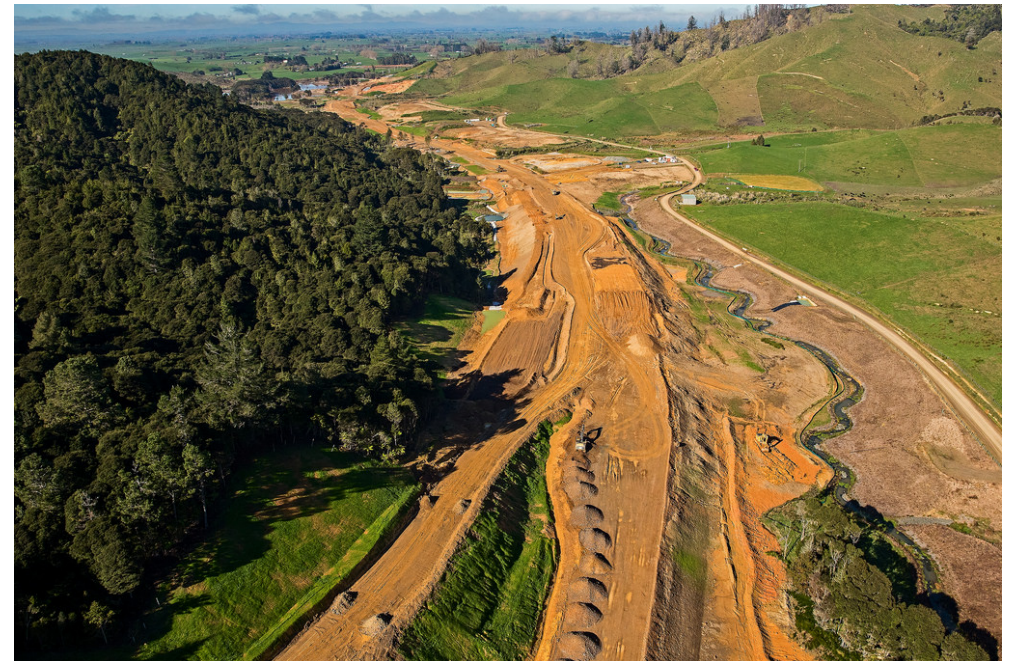
Waikato expressway- Grahams Valley Huntly
