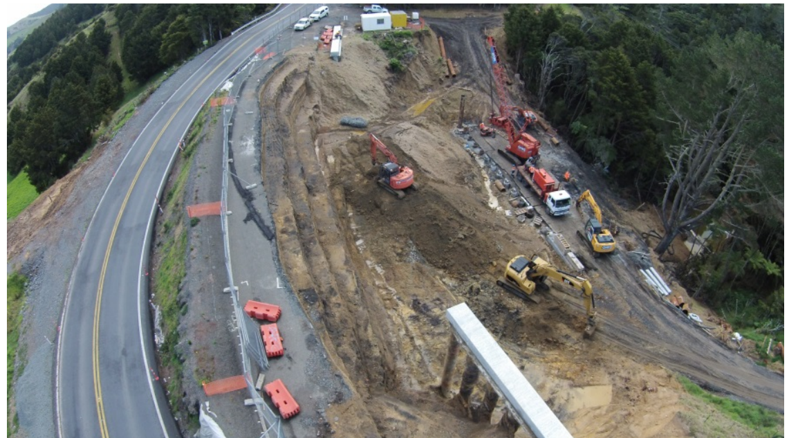
Significant projects are underway on the corridor
