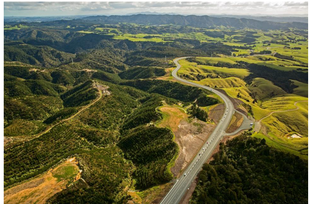
Significant safety improvements have been undertaken on the Brynderwyn Hills
