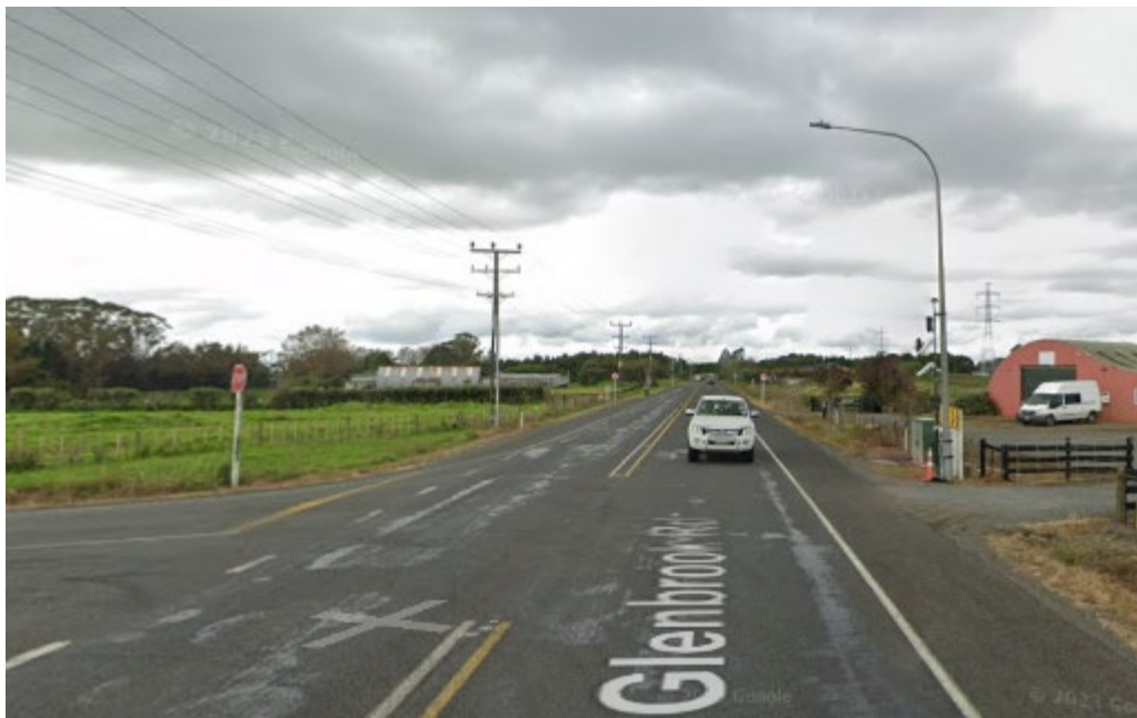
Installation location of second camera
