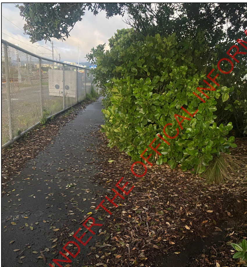
Figure 16: Poor vegetation clearance along the existing path to the north of the interchange
