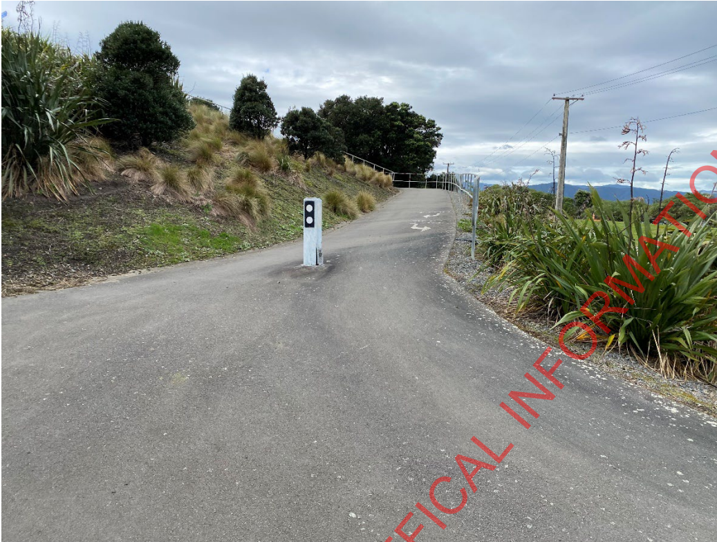
Figure 18: Ramp from connecting pathway to Hutt Road with potential speed issue.
