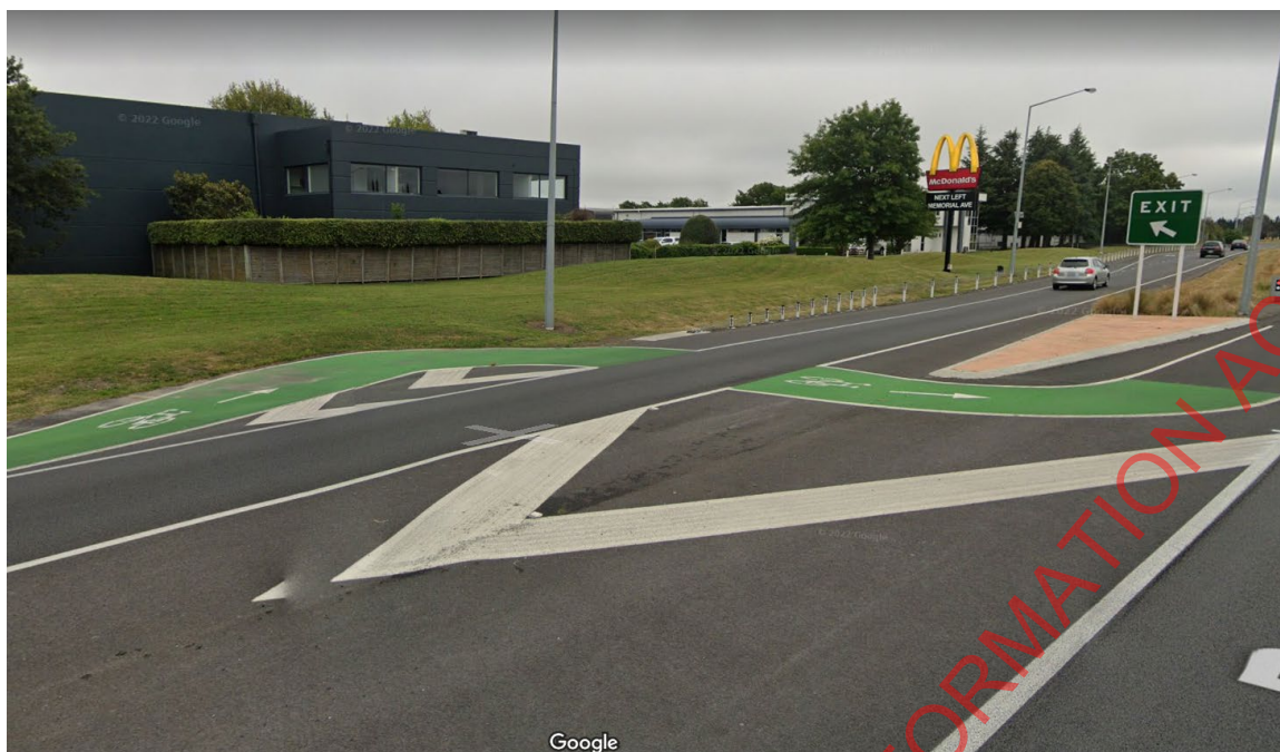
Figure 10: Example of bicycle crossing at off ramp at 90degrees to the movement
