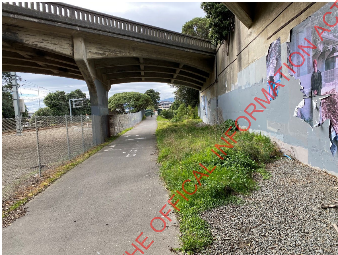
Figure 20: Existing intimidating environment below underpass
