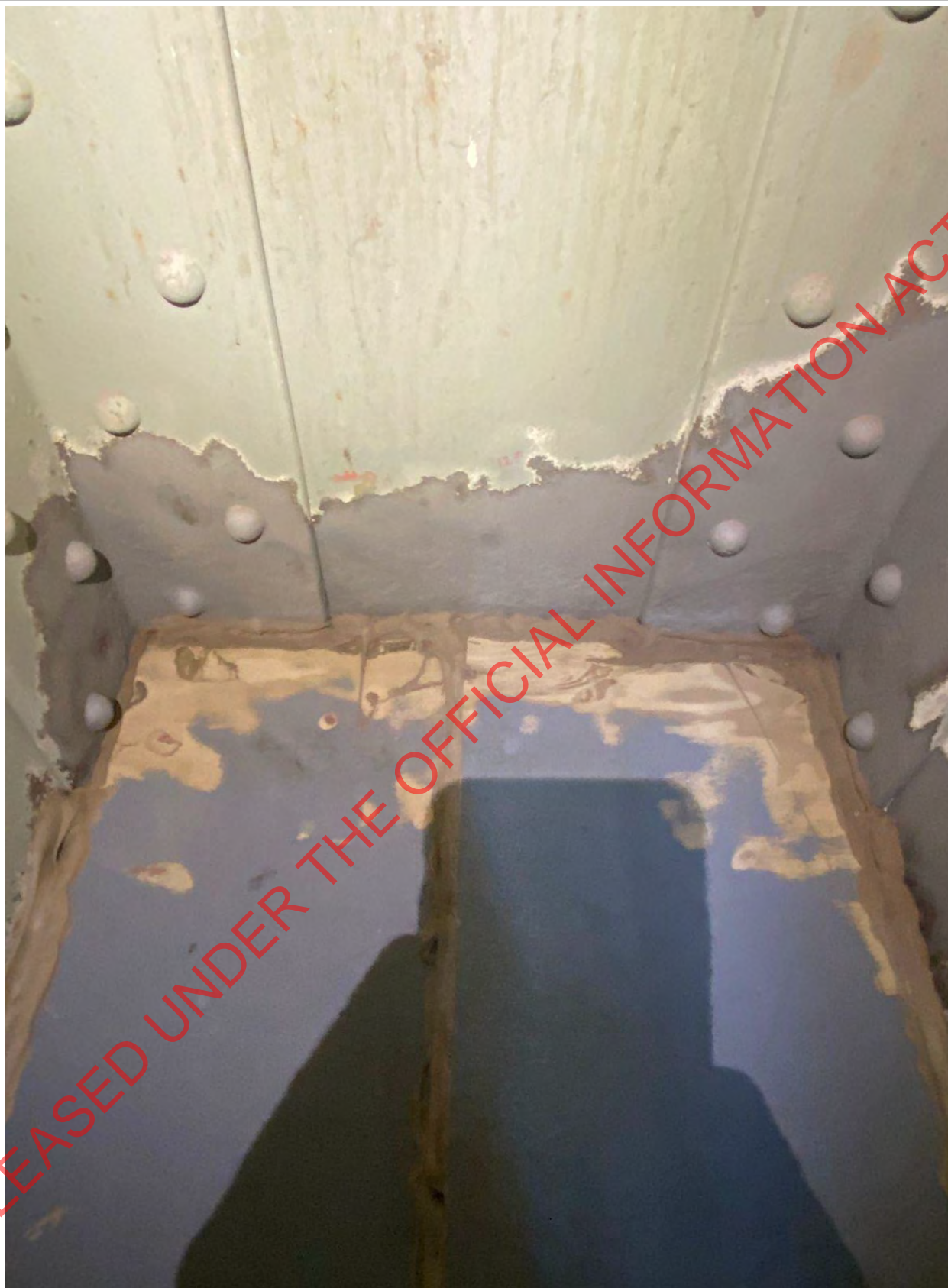
Area of corrosion following abrasive blasting
