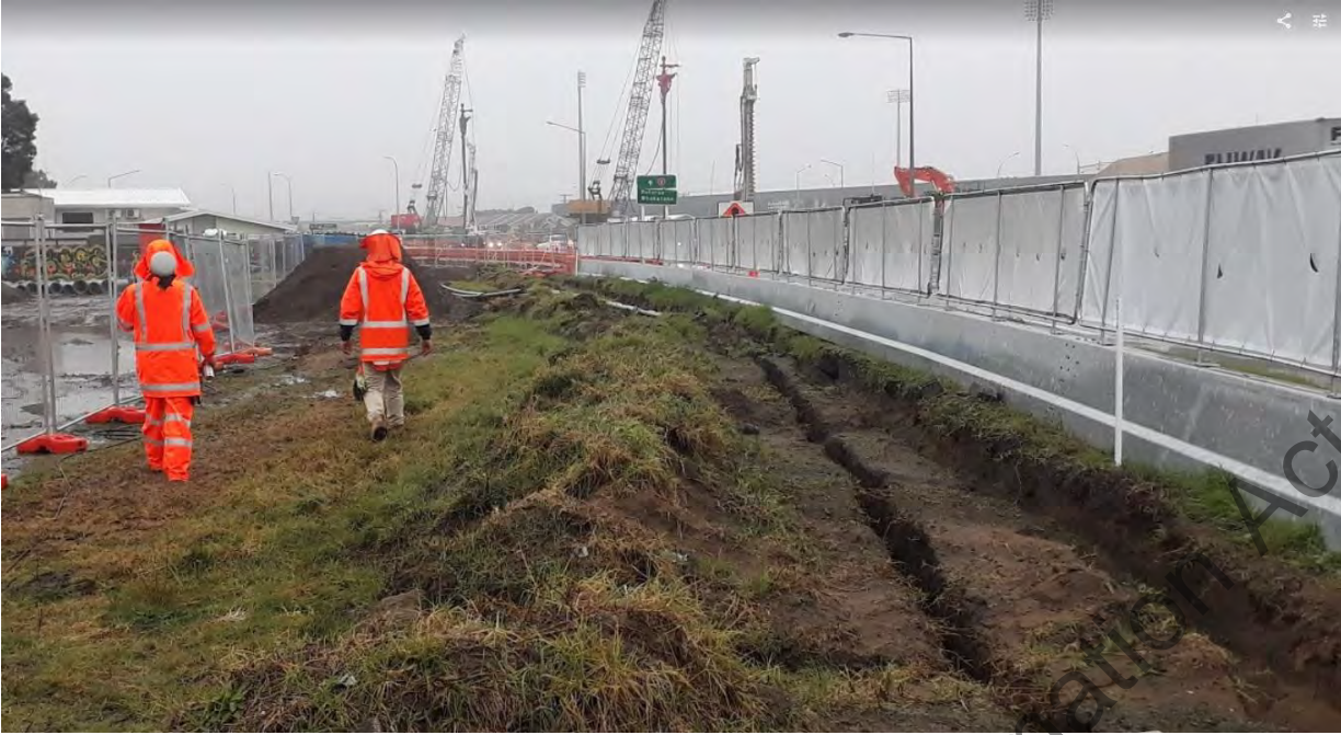
Relocation of Chorus network Trial Embankment area (area 2E)
