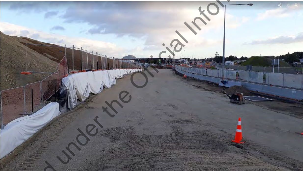
Canyon Subgrade (NB mainline) in triangle
