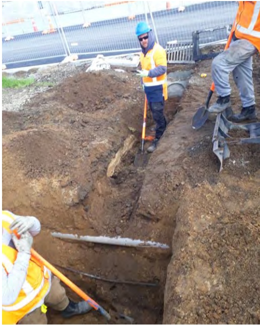
Hand & Hydro excavation works in 2A & 2C
