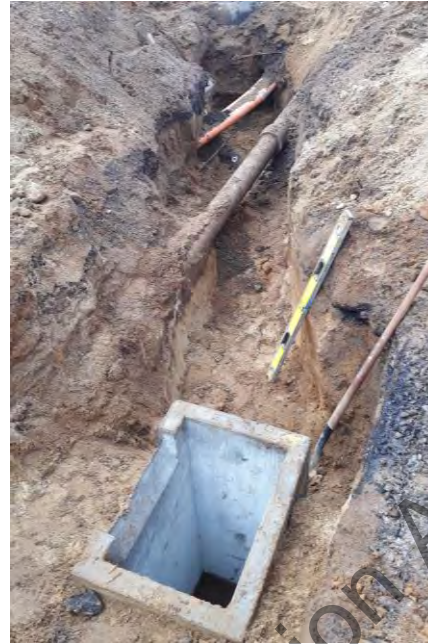
Hand & Hydro excavation works in 2A & 2C
