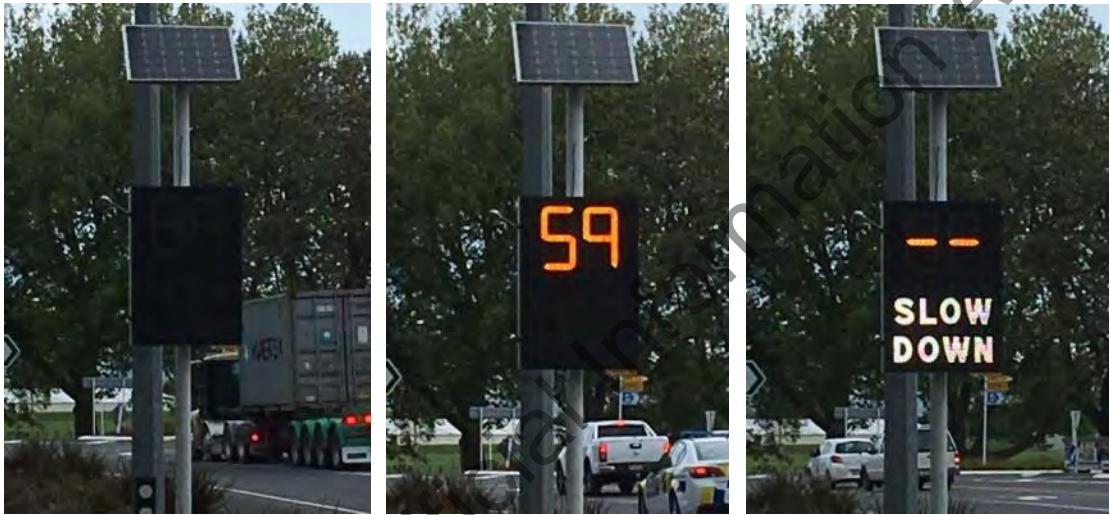
Figure 1 – Dynamic sign showing speed and slow down message
