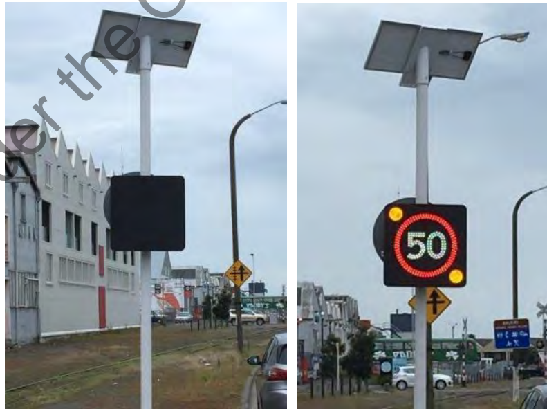
Figure 2 – Dynamic sign reinforcing speed limit with wig-wag signals
