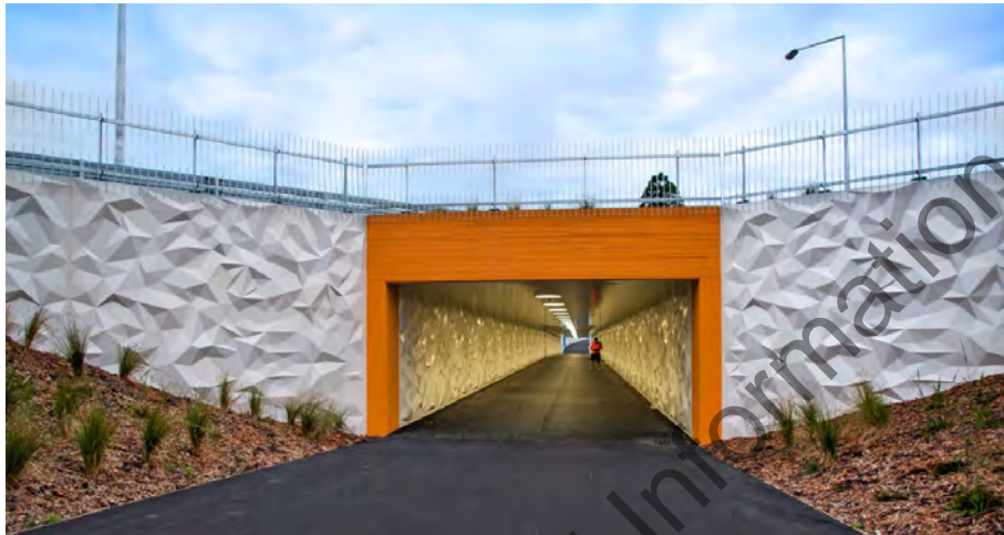
Figure 6: Photo of SH1 Russley Road/Harewood Road underpass
