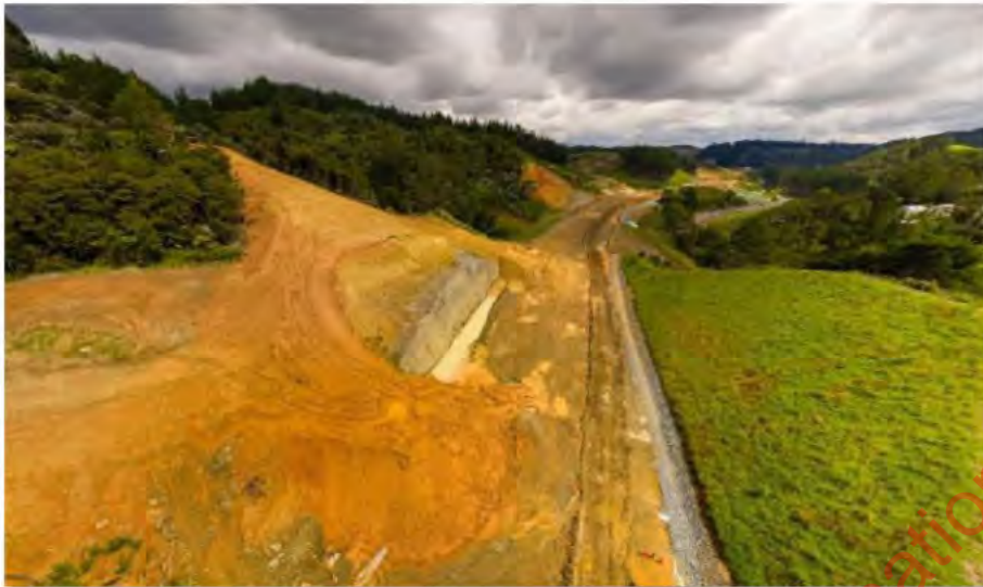
CS15A View in northern direction (Source: Landslide update 2020.45, Photo Date unknown)
