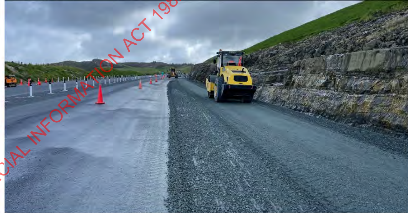
19/09/22 CS3 - Compacting AP40 Stage 2 on southbound shoulder, looking north
