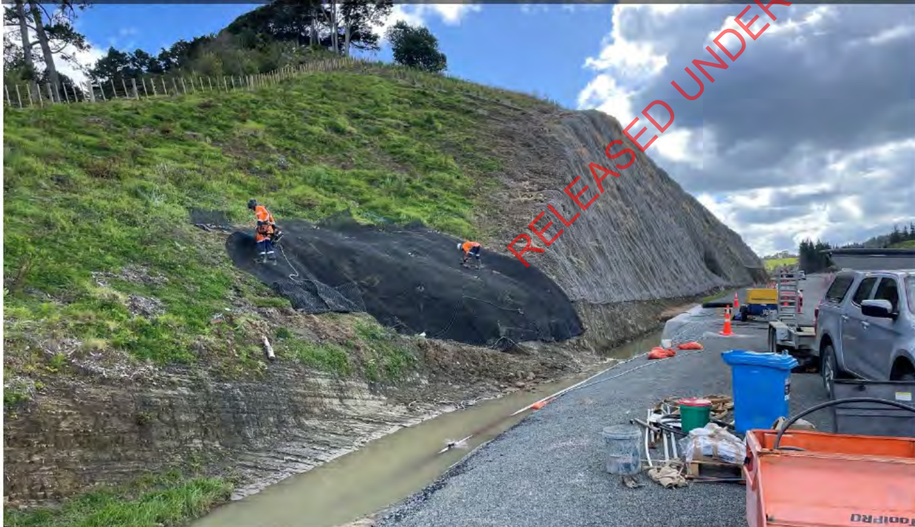
19/09/22 CS16D slip remedial works, looking north
