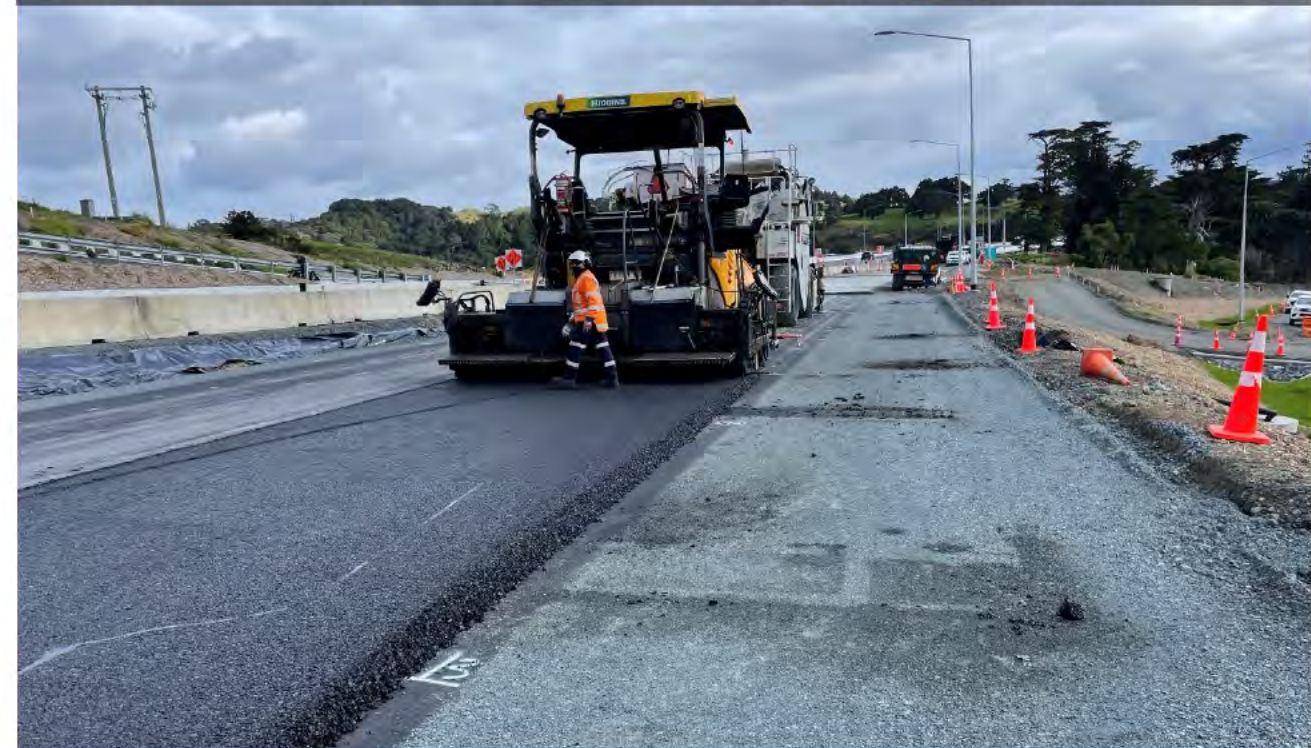
19/09/22 S7 - Laying AC20 on southbound lanes, looking north
