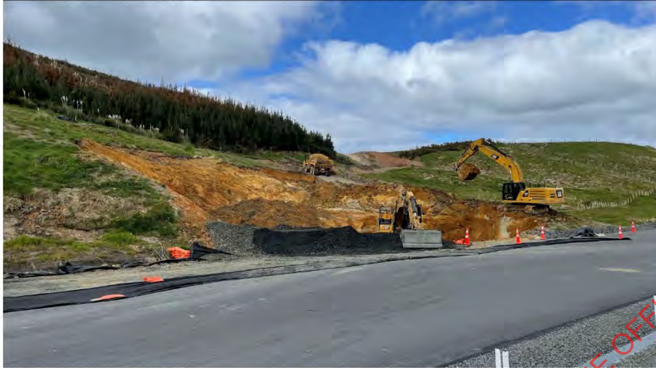
15/09/22 CN12 slip remedial works, looking east
