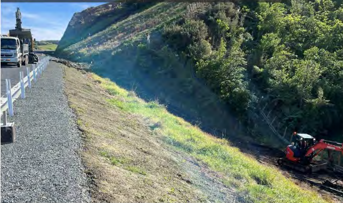
CS4: Remedial work on grass lined swale, ch.58500 (looking north)
