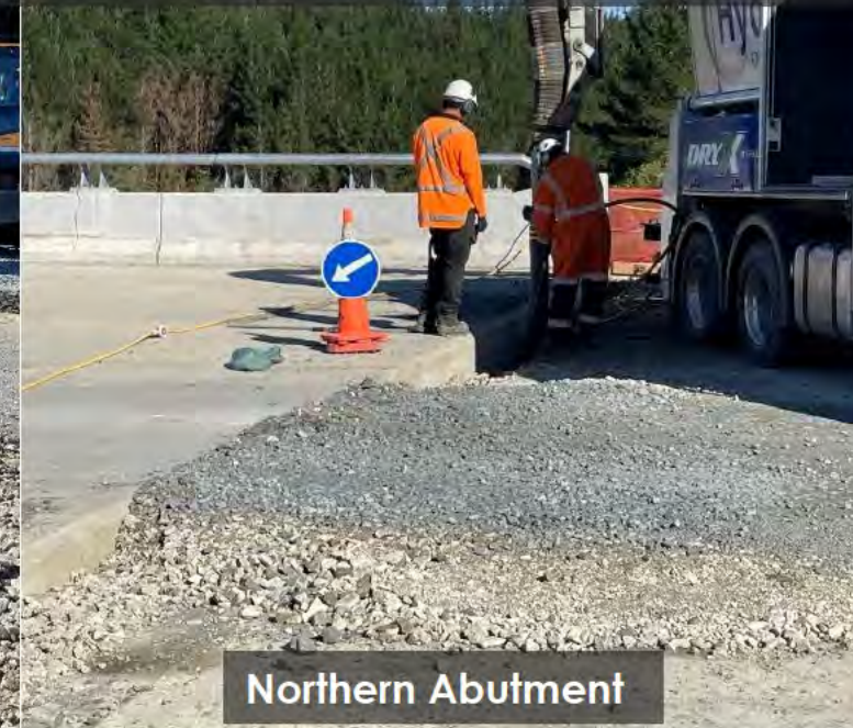
Watson Road Bridge: CJV excavating gravel pads either side of bridge deck, ch.63300 (looking north)
