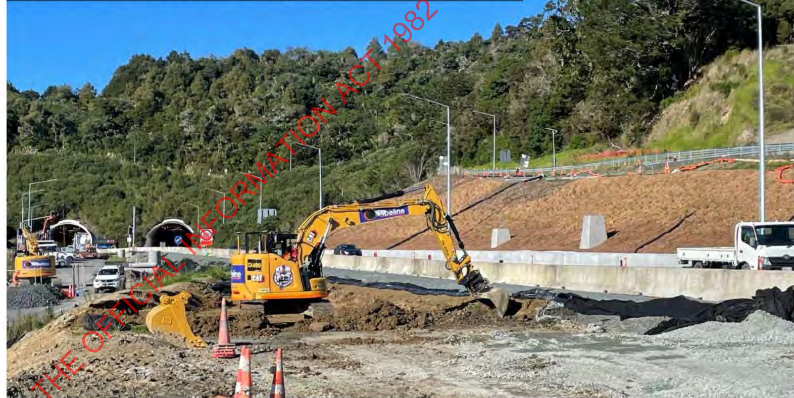
Southern tie-in: Existing subgrade removal for pavement construction, ch.65000 (looking south)
