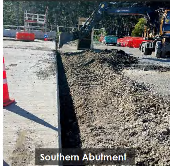
Watson Road Bridge: CJV excavating gravel pads either side of bridge deck, ch.63300 (looking north)
