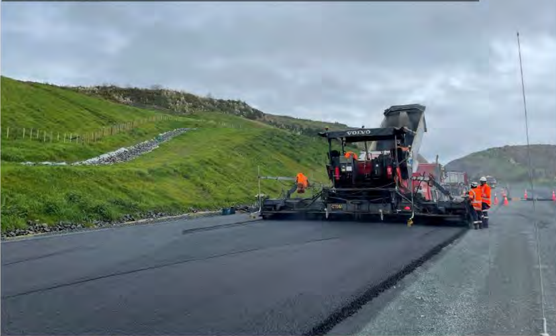
CN5: AC20 construction on southbound lane, ch.53500 (looking south)
