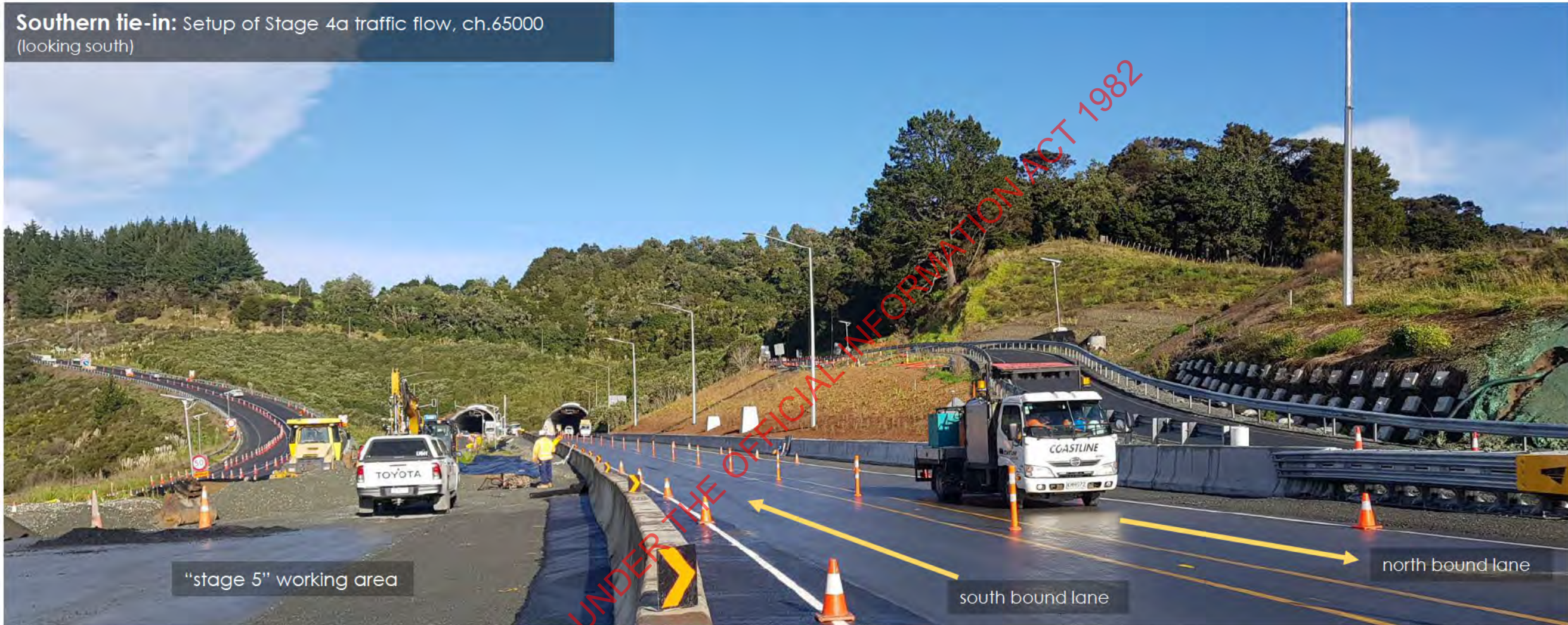
JHT: AP14 placed, compacted for median chicane, ch.65000 (looking south)
