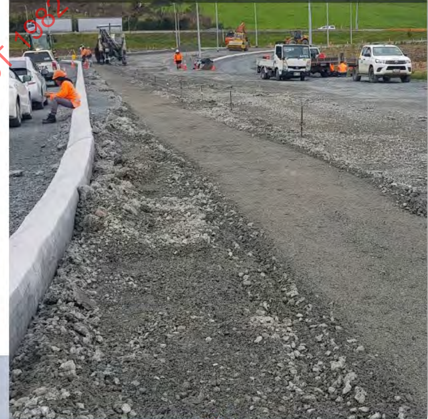
ROA: Roundabout median island kerb re-construction, 47000 (looking east)
