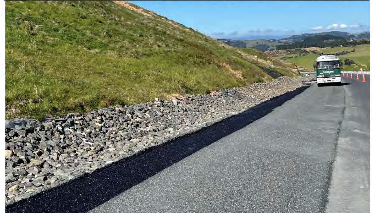
5/8/22 CS2 ch 57500 Prime/chipseal on southbound shoulder
