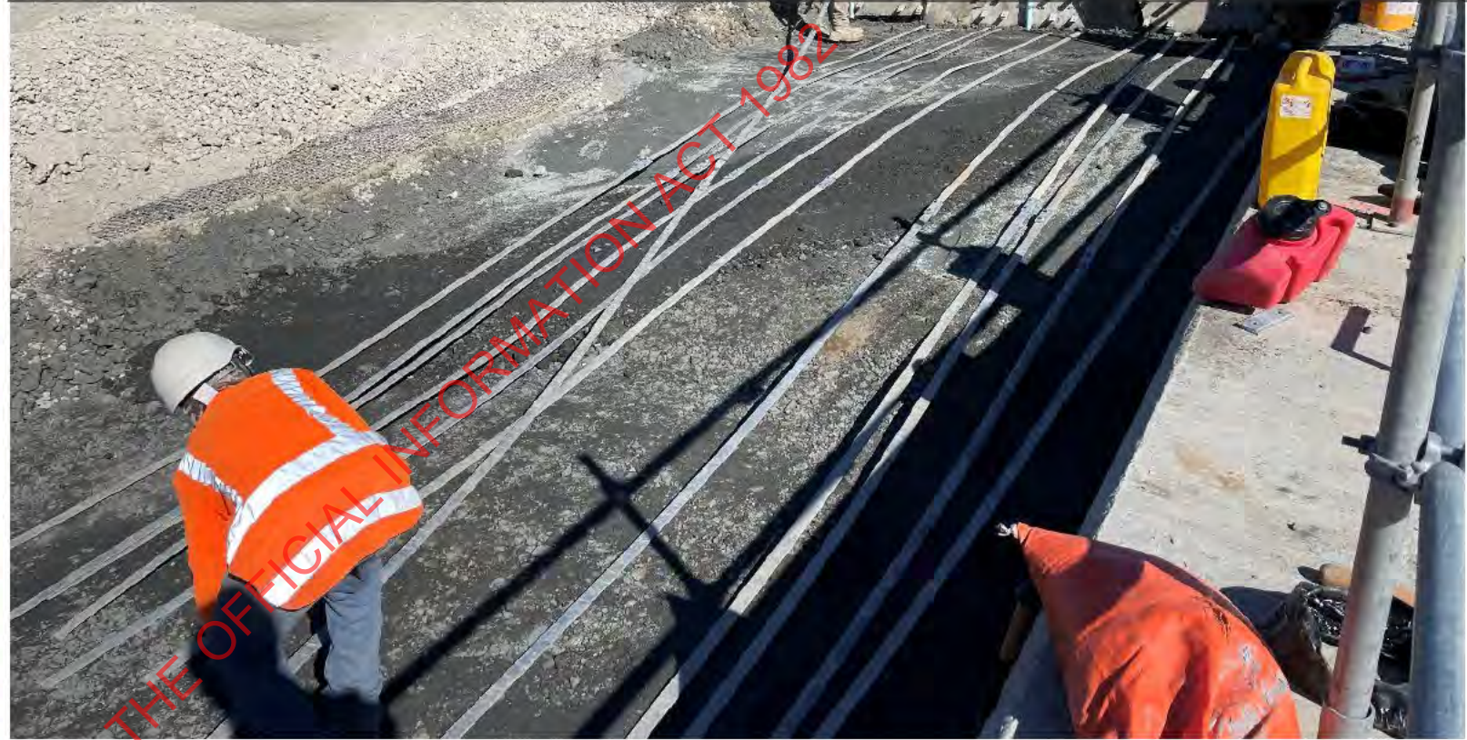
5/8/22 CS2 ch 57500 Prime/chipseal on southbound shoulder
