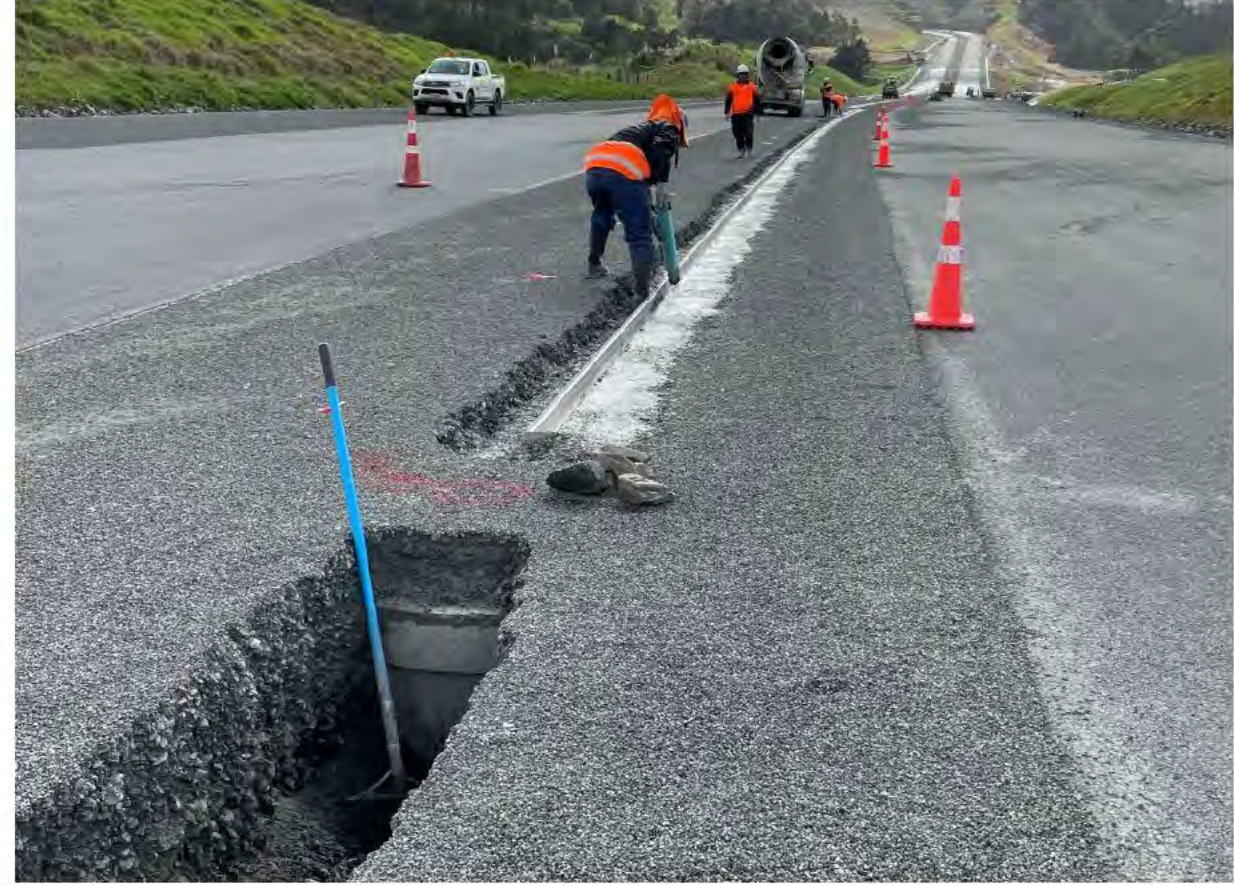
29/7/22 Installing Median Drains CN5
