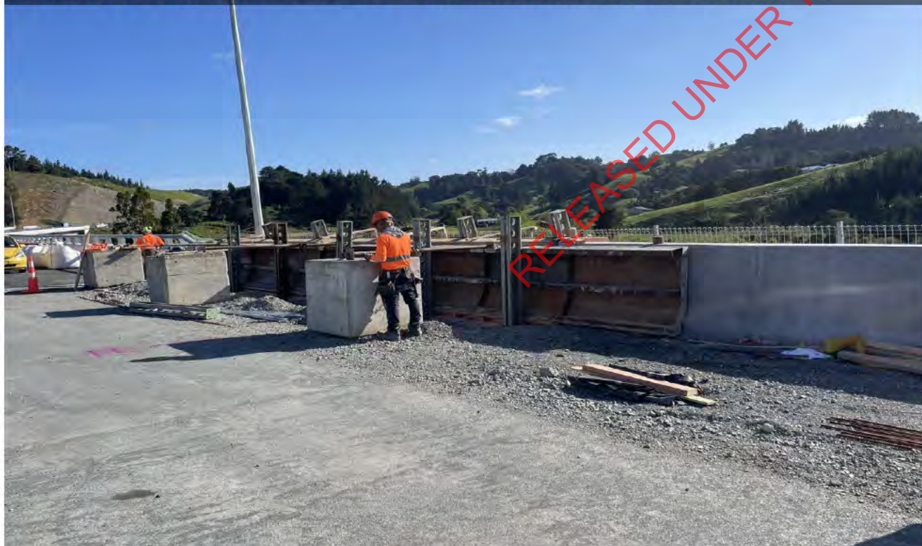
27/10/22 Cast insitu concrete barrier transition at Puhoi Bridge
