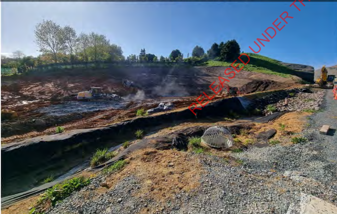
27/10/22 WM5 Lime stabilisation of permanent pond
