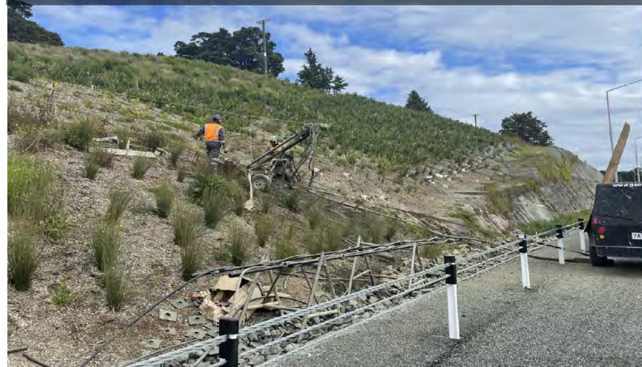
28/10/22 Soil Nail installation nearing completion at Okahu Viaduct (looking Northbound)
