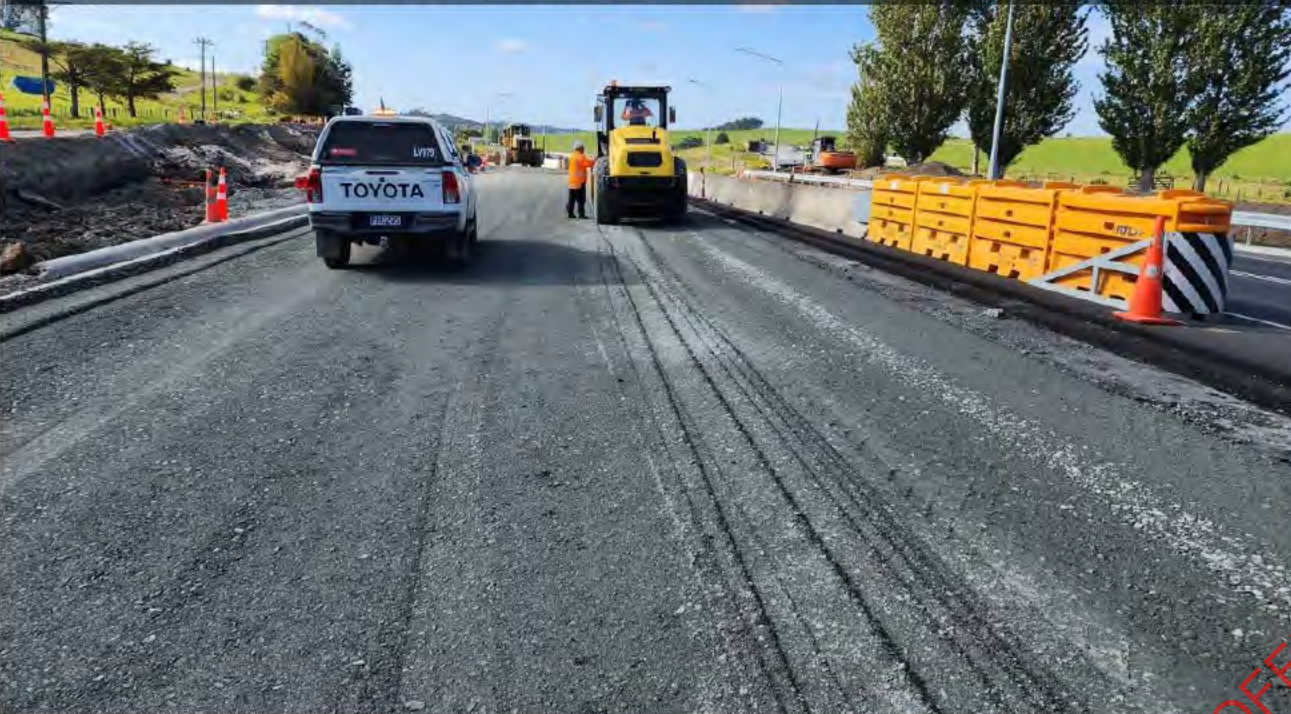
27/10/22 Pavement Construction Western Leg by Goatley Rd (SB)
