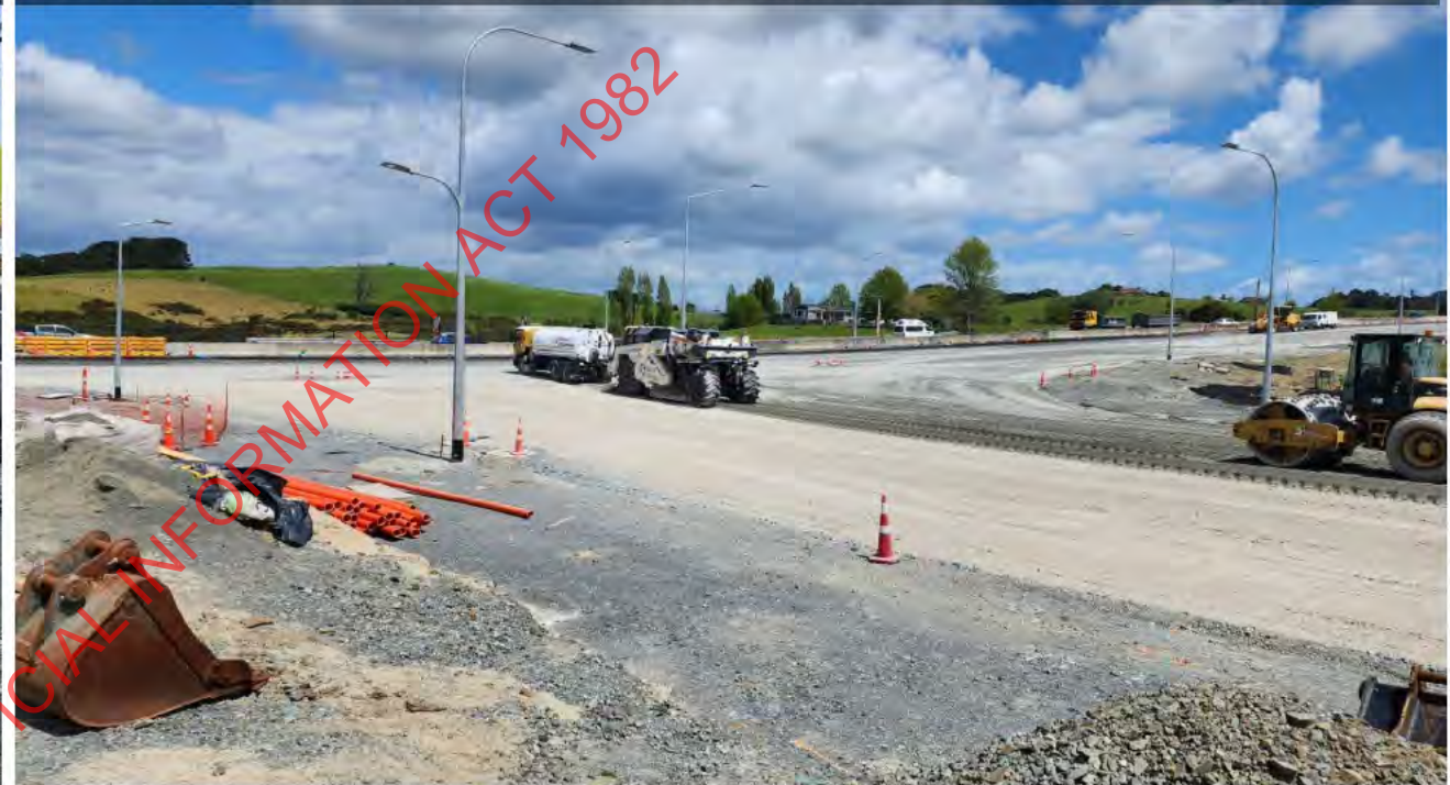
26/10/22 Pavement Construction at MRLi (towards SH1)
