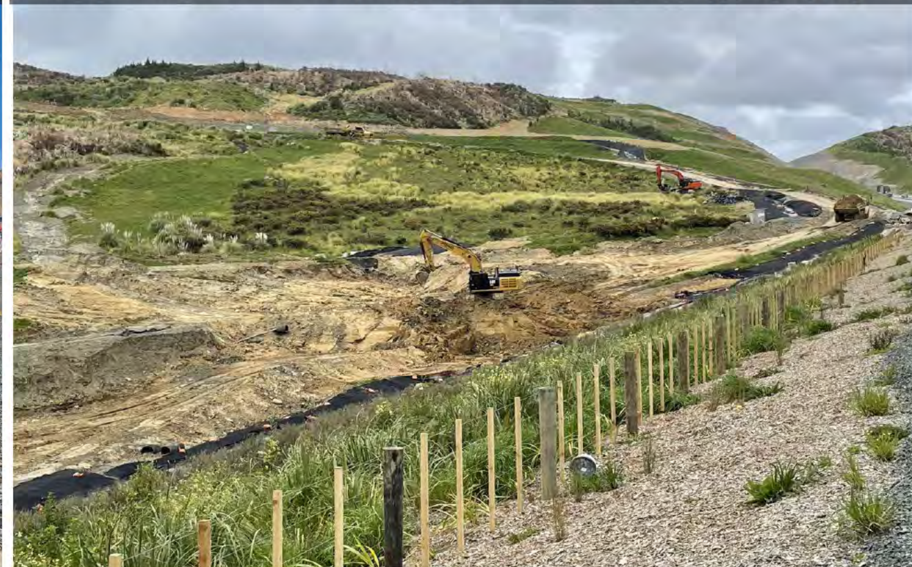
25/10/22 Large earthworks/shaping around Brokeback (looking SB)
