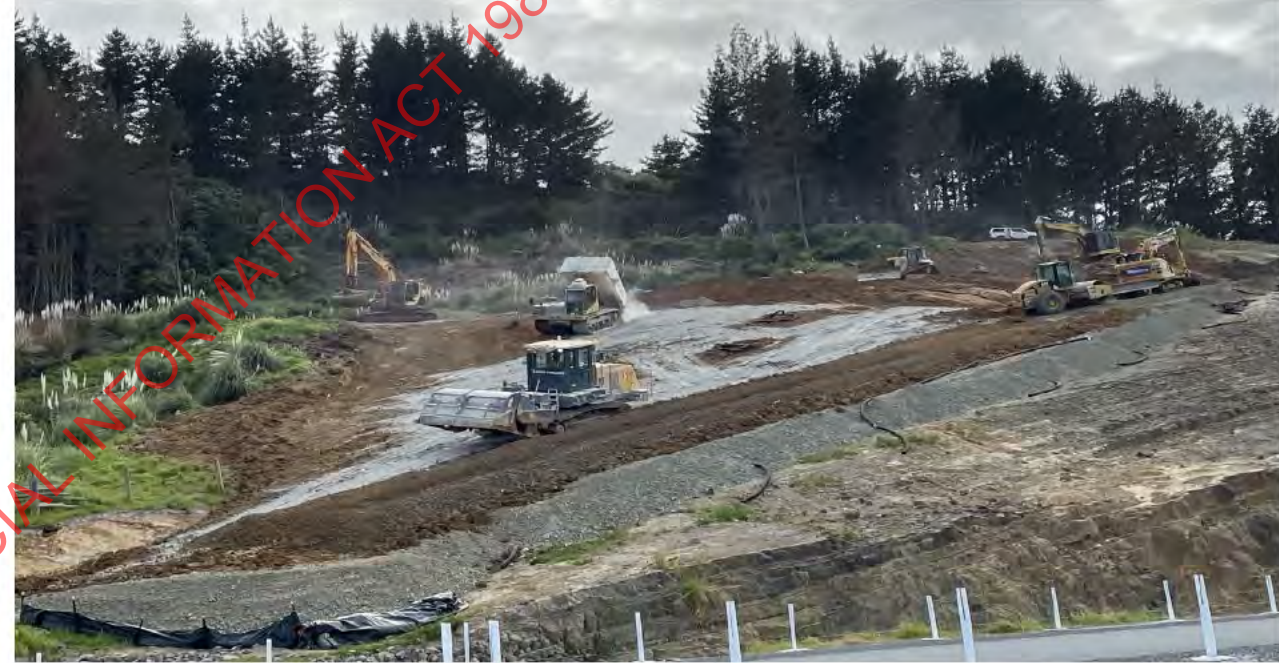
28/10/22 Soil Nail installation nearing completion at Okahu Viaduct (looking Northbound)
