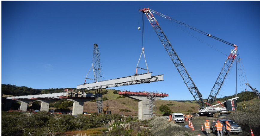
Photo of Arawhiti ki Ōkahu (Ōkahu viaduct)
