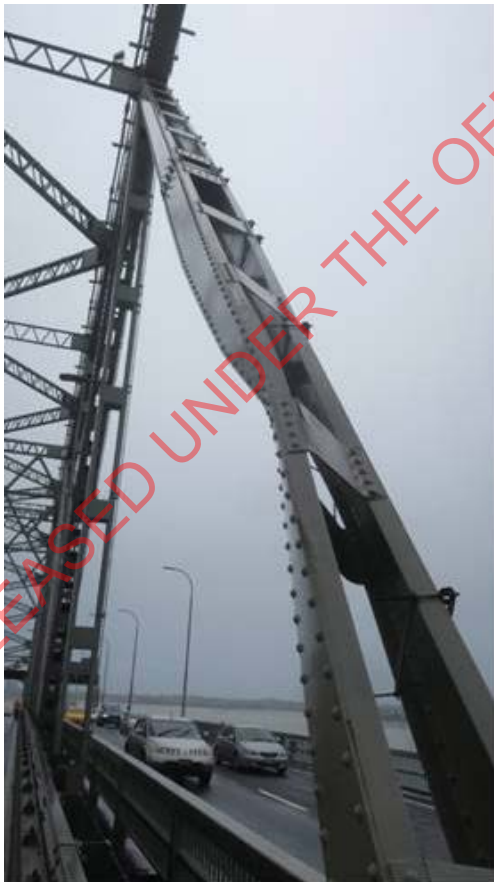
Caption: The bridge strut bent out of shape after being hit by a truck on the Auckland Harbour Bridge
